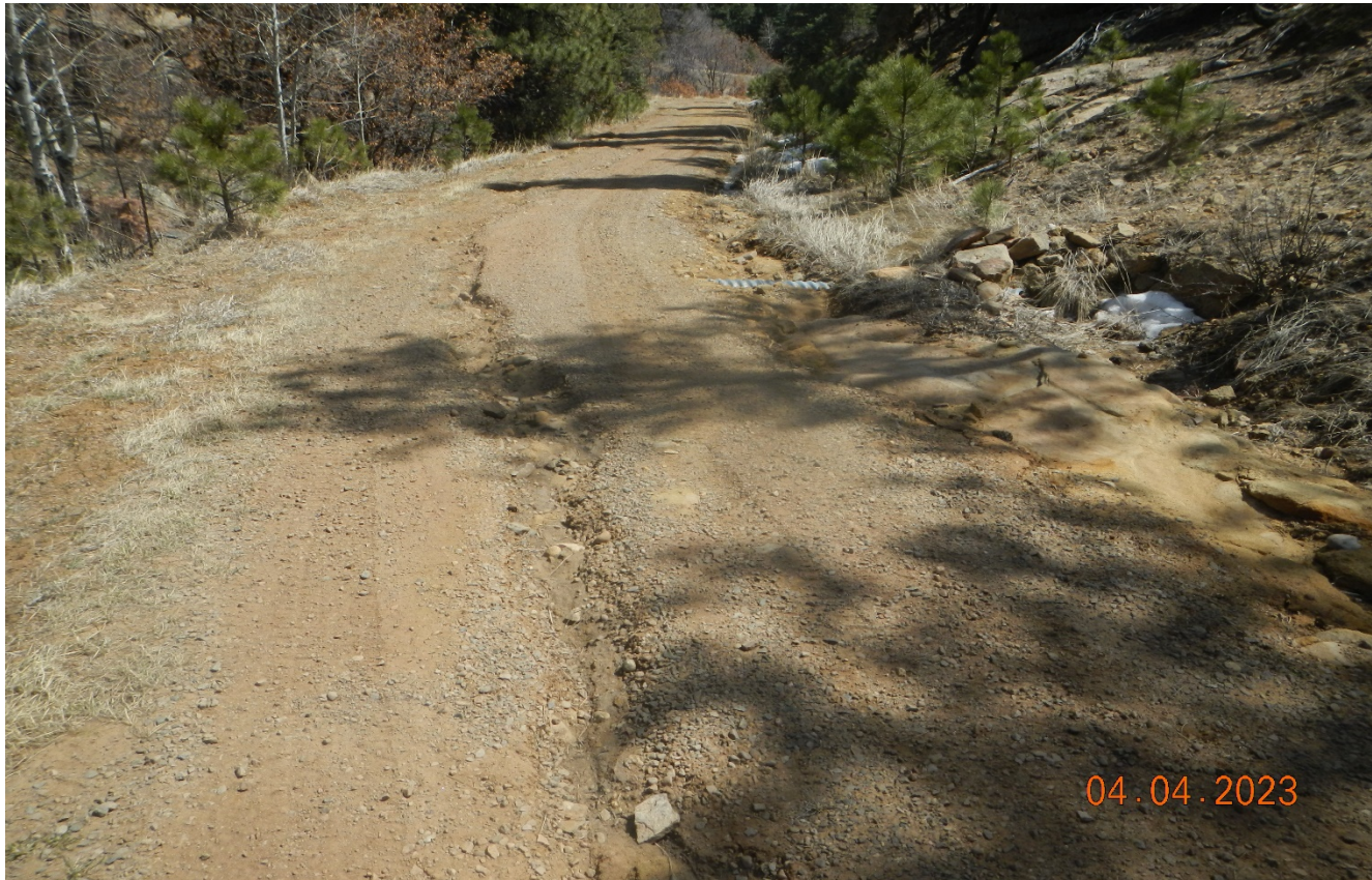
Photo 1. Facing east along the access road. There is erosion occurring along the road and stormwater is not being directed toward the culvert.
