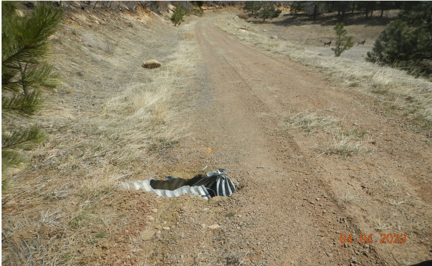
Photo 2. Further down the access road is a damaged culvert that will need to be repaired.
