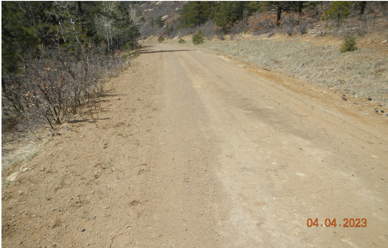
Photo 1. Facing southwest along the main access road. Areas of erosion along the road have been graded out.
