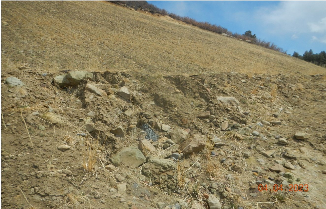
Photo 8. Facing northeast at west side of the location. There are some areas of erosion that should be repaired with BMP's to control further erosion.
