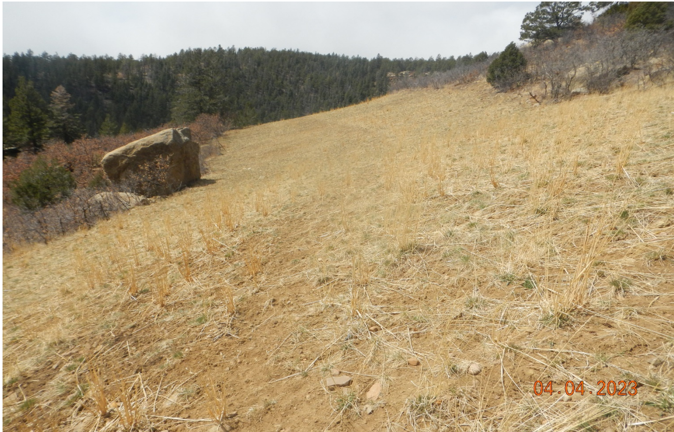
Photo 2. Facing southwest at the beginning of the reclaimed access road. The perennial vegetation appears to be establishing along the reclaimed road.
