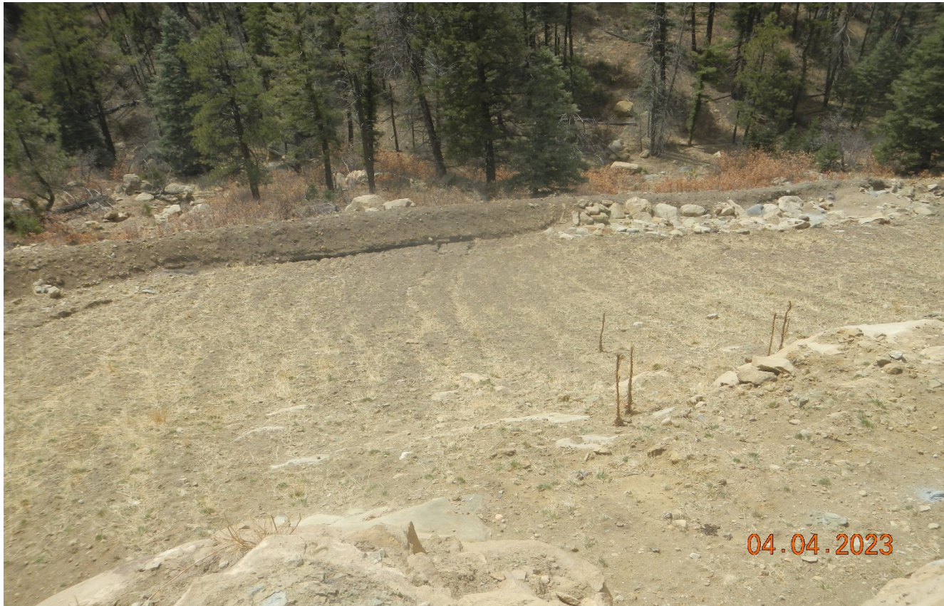
Photo 7. Facing down toward the bottom of the location. The berm at the bottom appears to need some maintenance due to erosion.
