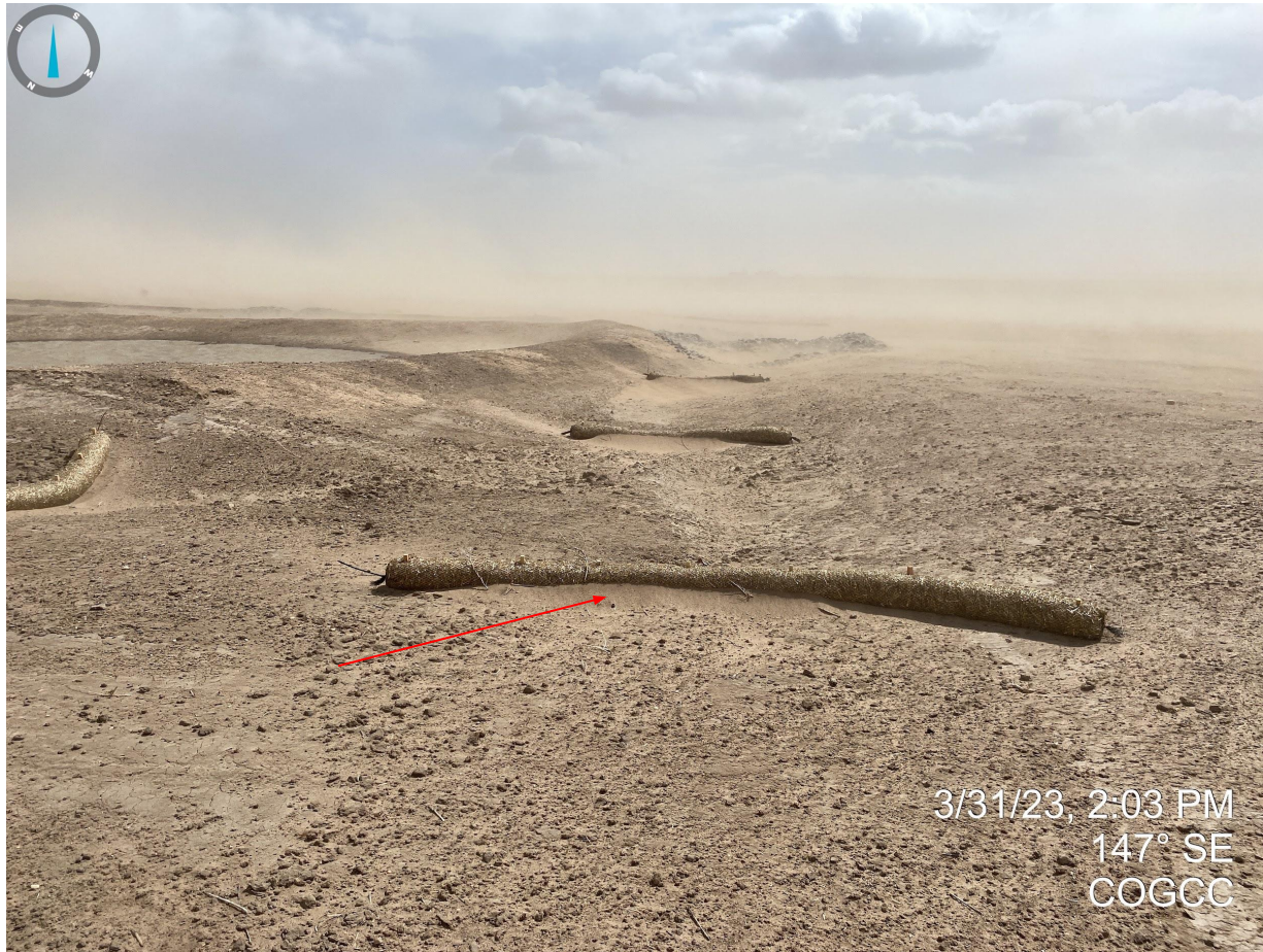
Photo 10. Facing southeast from the northwest corner of the location. Straw wattles will need to be maintained to ensure they are properly functioning in the future.
