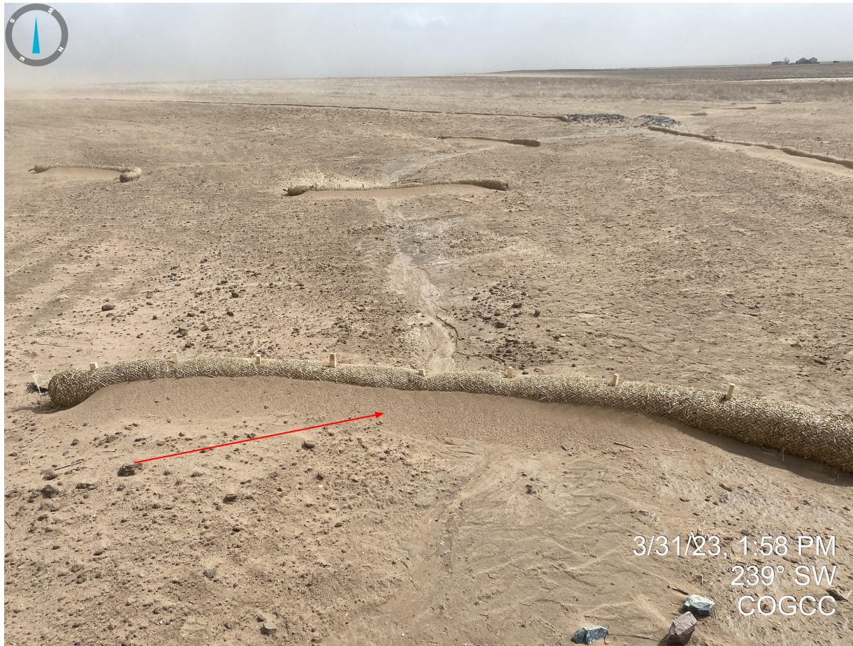
Photo 3. Straw wattles placed as check dams within the eroded areas. Blow sand from high winds have accumulated within the straw wattles and will require maintenance to ensure the BMPs are properly functioning.
