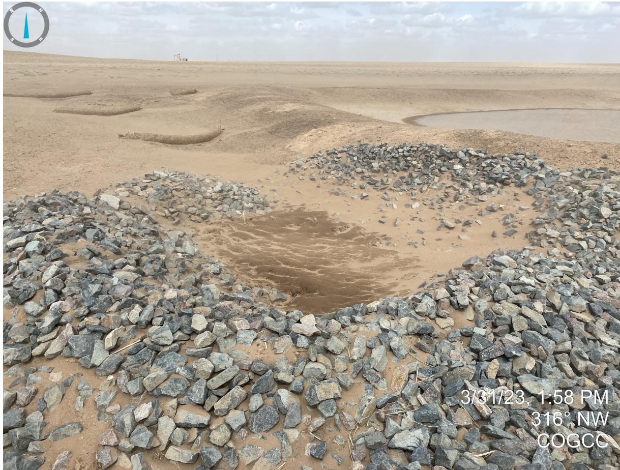
Photo 1. Sediment trap and straw wattles installed in the area previously experiencing erosion issues. It appears the Stormwater BMPs will be sufficient at controlling and managing stormwater for this location.
