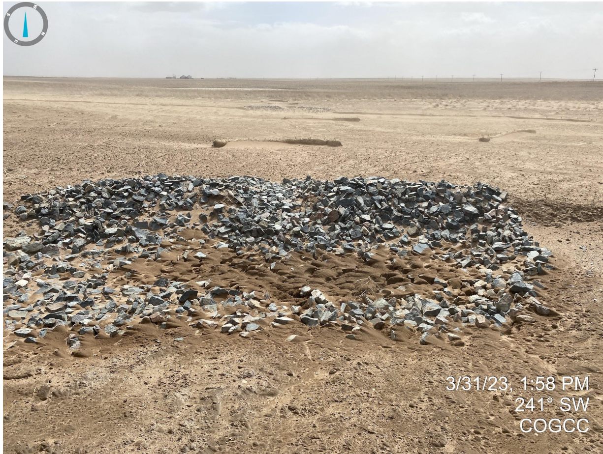
Photo 4. Sediment trap installed at the southern end of the location appears to have been stabilized with rip rap material.
