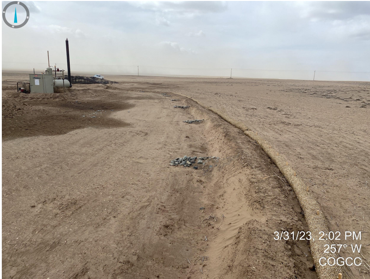
Photo 8. Berm and ditch BMPs appear to have been compacted and additional BMPs have been implemented (check dams within ditch and straw wattles placed on the exterior portion of the berms).
