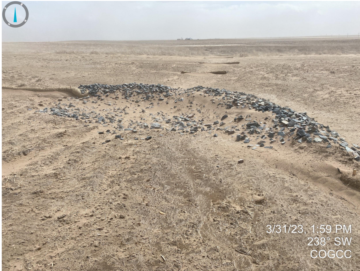
Photo 5. Additional sediment trap placed within the recently reclaimed portion of the location.
