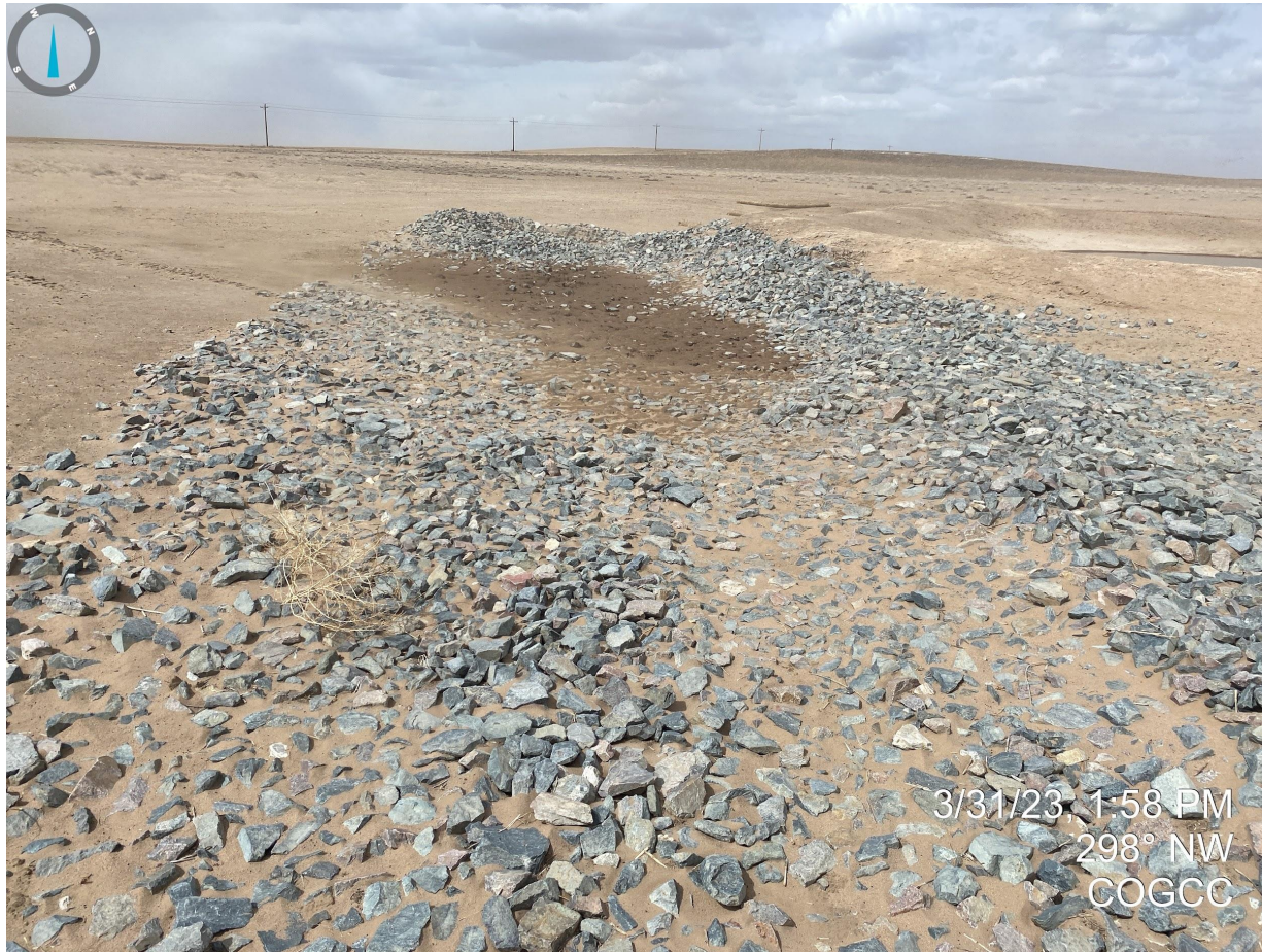
Photo 2. Rip rap structure/water bar placed at the entrance to the pad.
