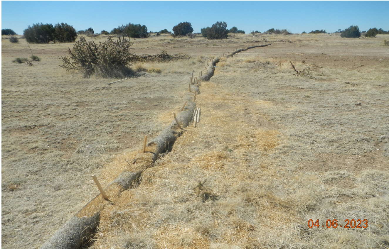
Photo 5. The perimeter wattles are degraded and not functional.
