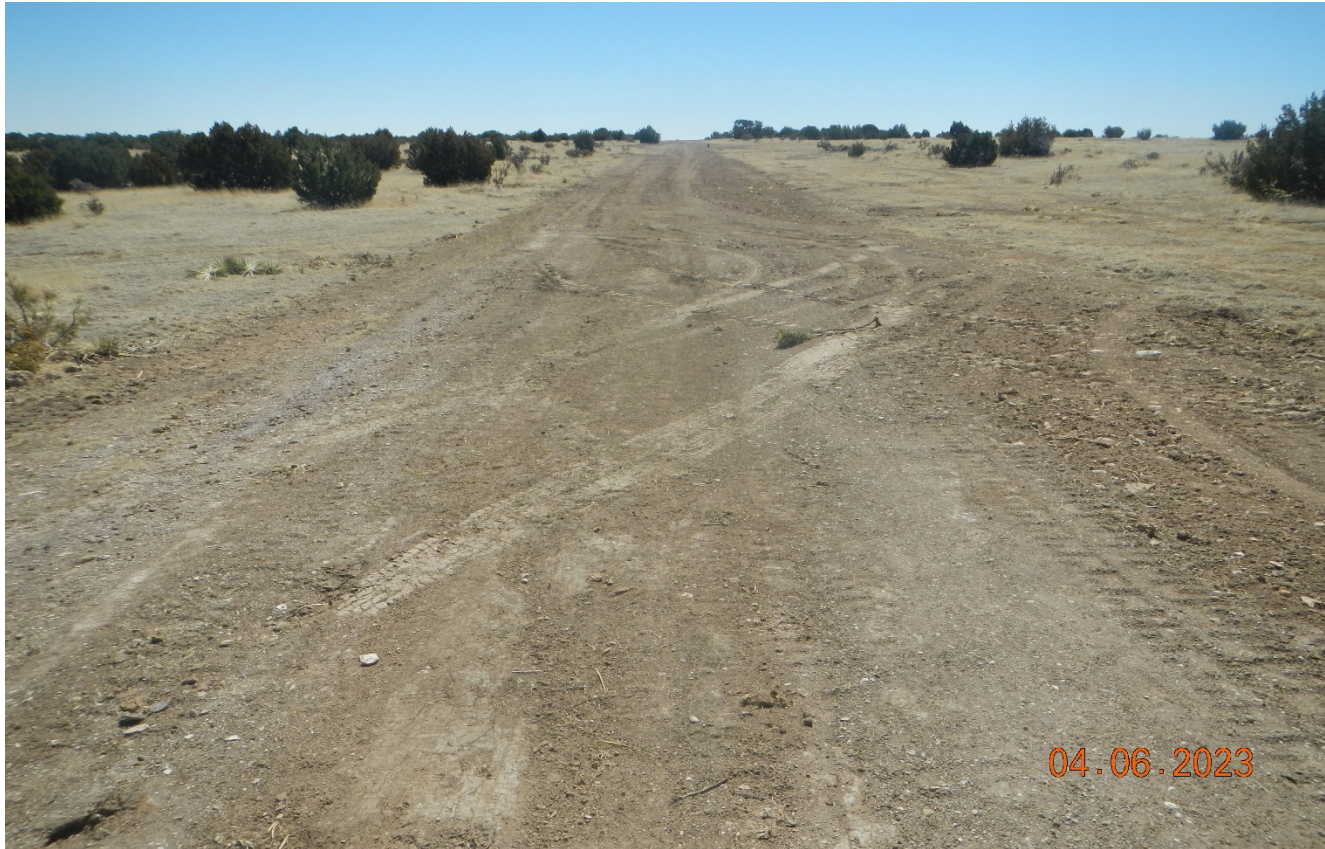
Photo 6. Facing south toward the flowline trenching disturbance. The piles of tree debris were mostly removed. All disturbed soils will need to be decompacted, seeded, and stabilized.
