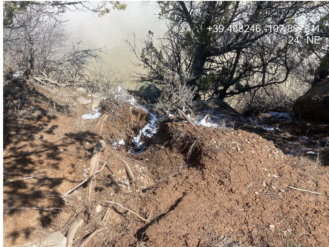
Photo 14. Photo taken from the northwest, shows where the access road ditch/western location perimeter ditch is causing offsite degradation to the north in the form of scouring, rills and a gully.
