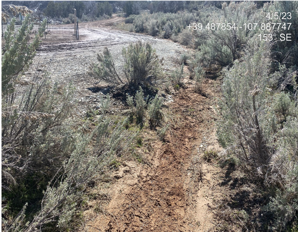
Photo 13. Photo taken from the northwest, shows where the access road ditch/western location perimeter ditch is causing offsite degradation to the north in the form of scouring, rills and a gully.
