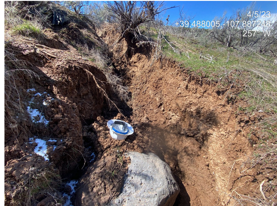
Photo 8. Photo taken from the northeast, behind the tank battery shows erosion degradation downslope of the ditch and outlet pictured in Photo 7.
