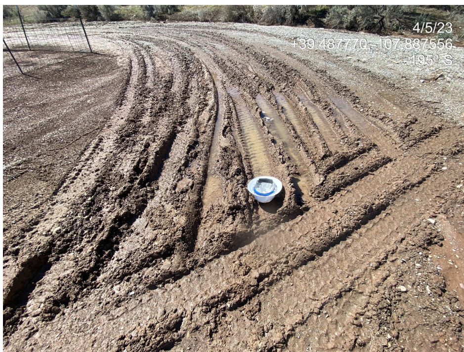
Photo 3. Photos show lack of stabilization of the working pad surface (ruts).
