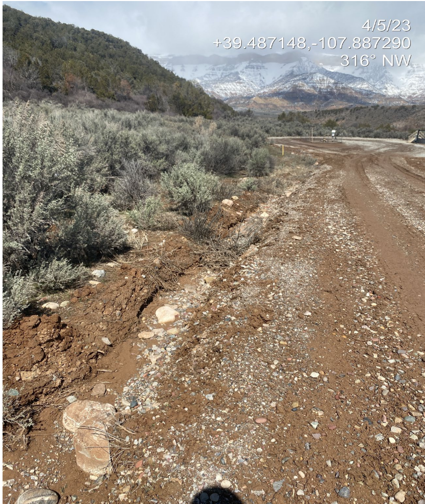
Photo 4. Photo shows the edge of the access road is unstable. The ditch is full of sediment and the ditch itself is eroding.
