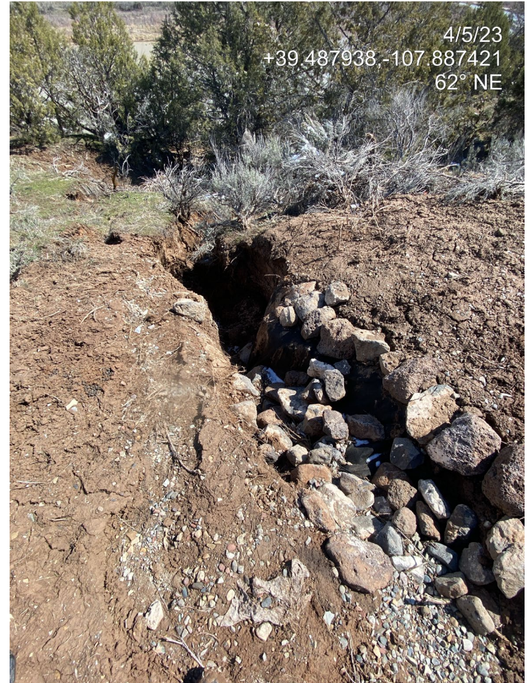
Photo 7. Photo taken from the northeast, behind the tank battery shows erosion degradation where a ditch leads to an outlet (arrow and left).
