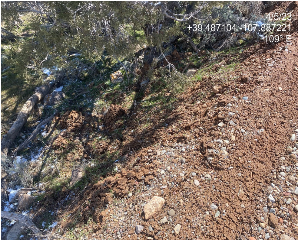
Photo 6. Photo shows the edge of the access road is unstable. Portions of the road are sloughing off.
