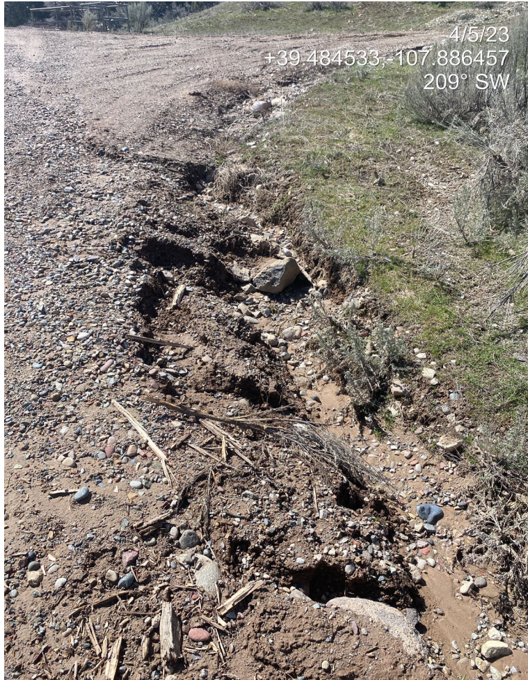
Photo 5. Photo shows the edge of the access road and ditch are unstable. Portions of the road are sloughing off.
