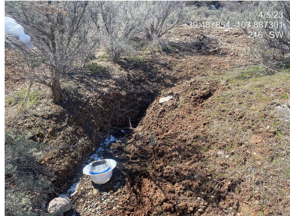
Photo 12. Photo taken from the northeast, behind the tank battery shows erosion degradation downslope of the ditch and outlet pictured in Photo 11.
