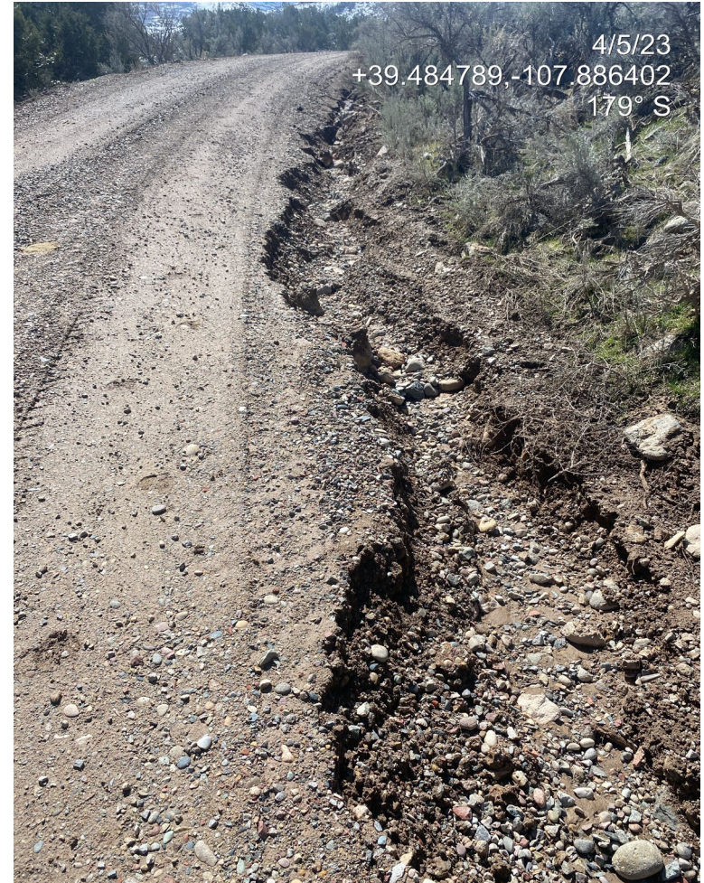
Photo 5. Photo shows the edge of the access road and ditch are unstable. Portions of the road are sloughing off.
