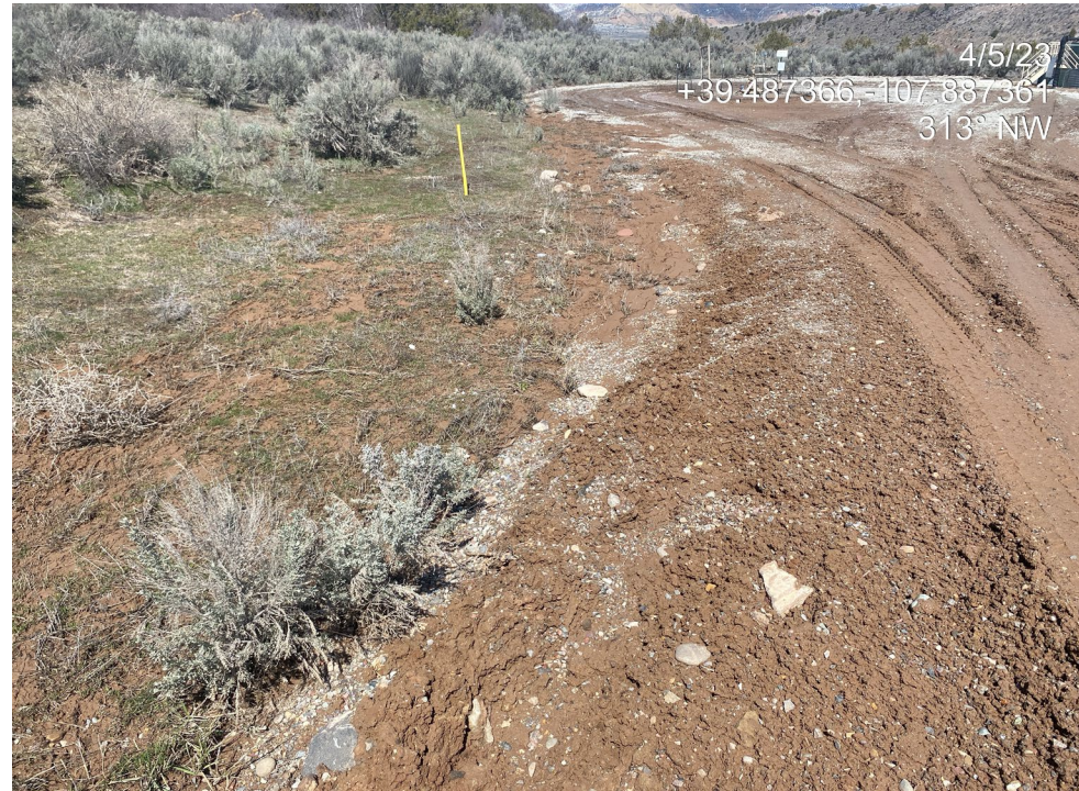
Photo 4. Photo shows the edge of the access road is unstable. The ditch is full of sediment and the ditch itself is eroding.
