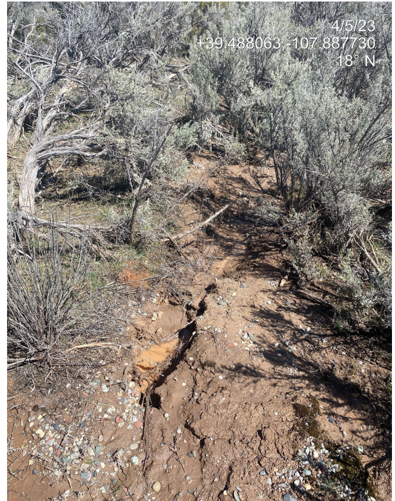
Photo 13. Photo taken from the northwest, shows where the access road ditch/western location perimeter ditch is causing offsite degradation to the north in the form of scouring, rills and a gully.
