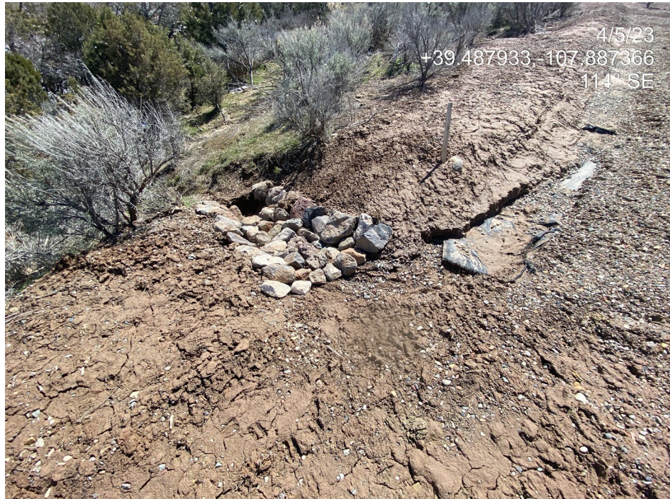
Photo 11. Photo taken from the northeast, behind the tank battery shows erosion degradation where a ditch leads to an outlet.
