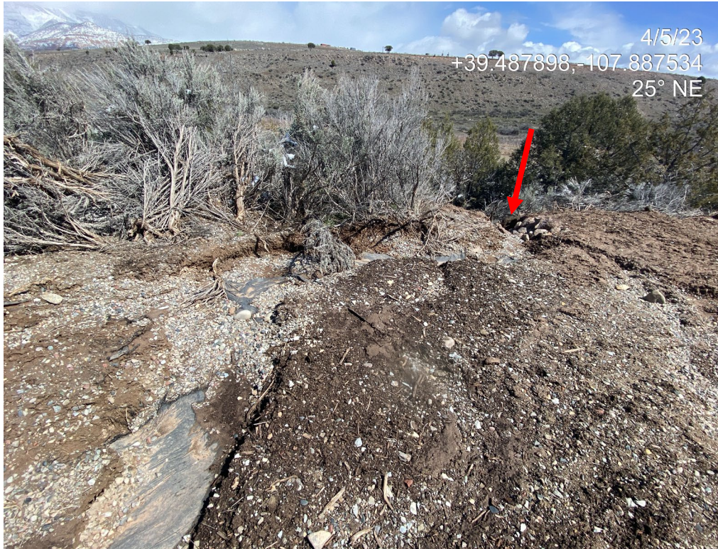
Photo 7. Photo taken from the northeast, behind the tank battery shows erosion degradation where a ditch leads to an outlet (arrow and left).
