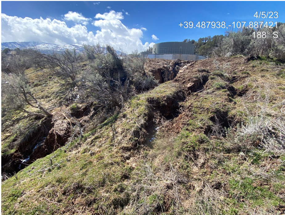
Photo 8. Photo taken from the northeast, behind the tank battery shows erosion degradation downslope of the ditch and outlet pictured in Photo 7.
