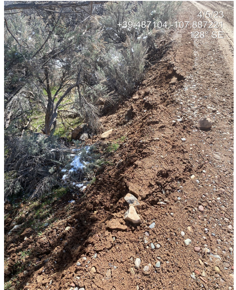
Photo 6. Photo shows the edge of the access road is unstable. Portions of the road are sloughing off.
