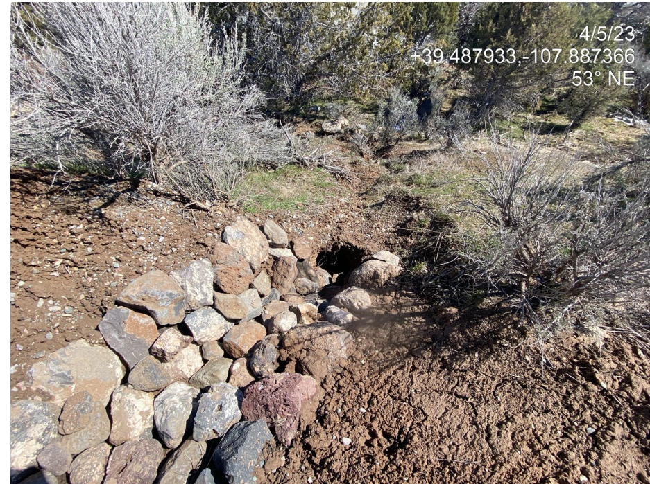
Photo 11. Photo taken from the northeast, behind the tank battery shows erosion degradation where a ditch leads to an outlet.
