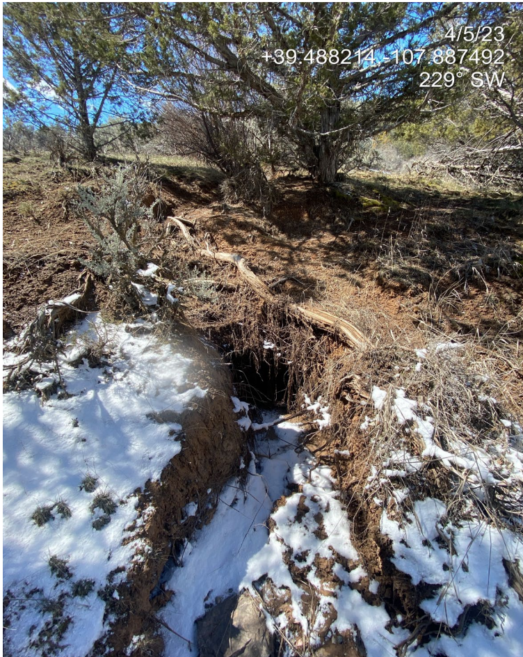
Photo 14. Photo taken from the northwest, shows where the access road ditch/western location perimeter ditch is causing offsite degradation to the north in the form of scouring, rills and a gully.
