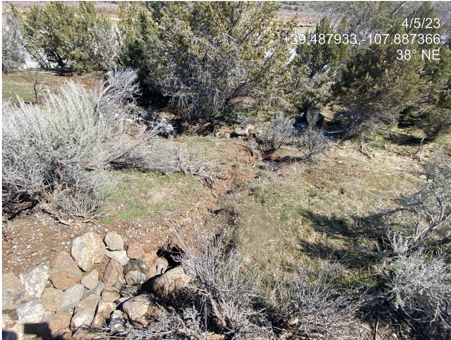
Photo 12. Photo taken from the northeast, behind the tank battery shows erosion degradation downslope of the ditch and outlet pictured in Photo 11.
