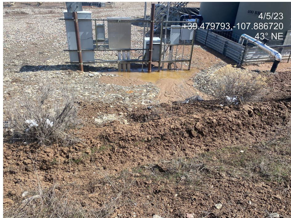
Photo 7. Photos show a berm at the south of the location is not stable. Rill erosion and sediment transport are evident.
