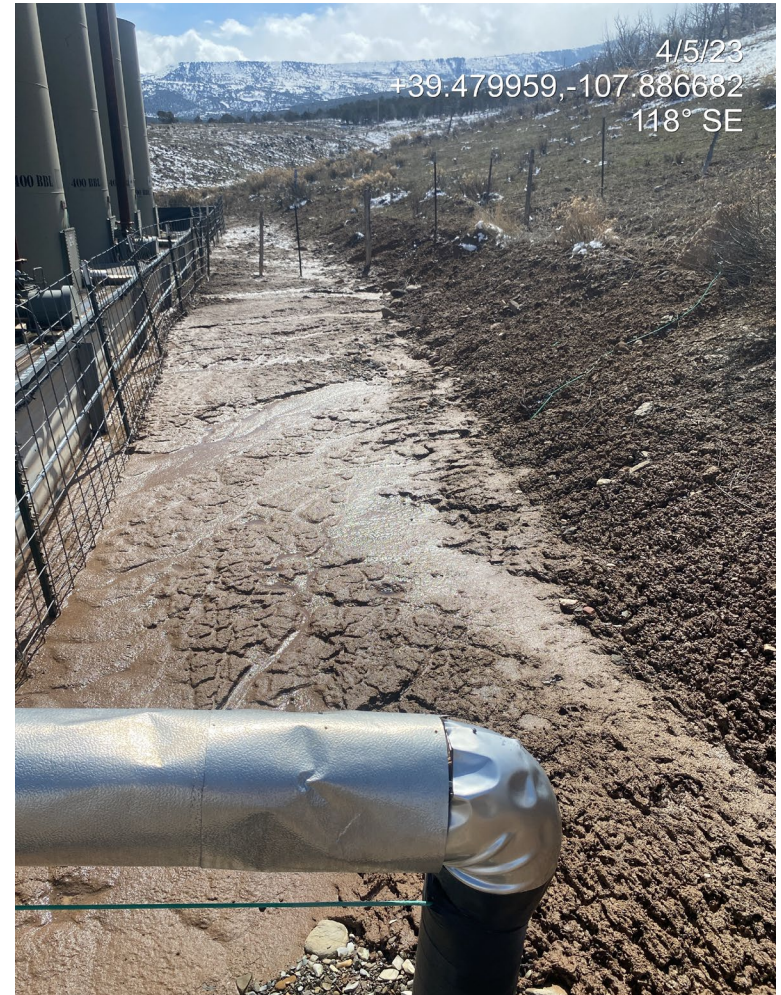
Photo 6. Photos show a berm at the south of the location is not stabilized. Rill erosion and sediment transport are evident.
