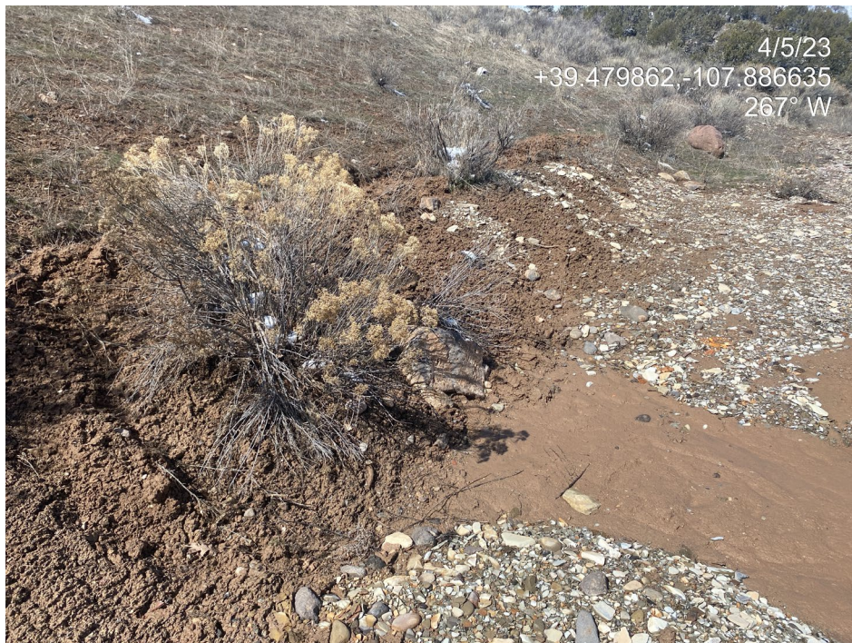
Photo 7. Photos show a berm at the south of the location is not stable. Rill erosion and sediment transport are evident.
