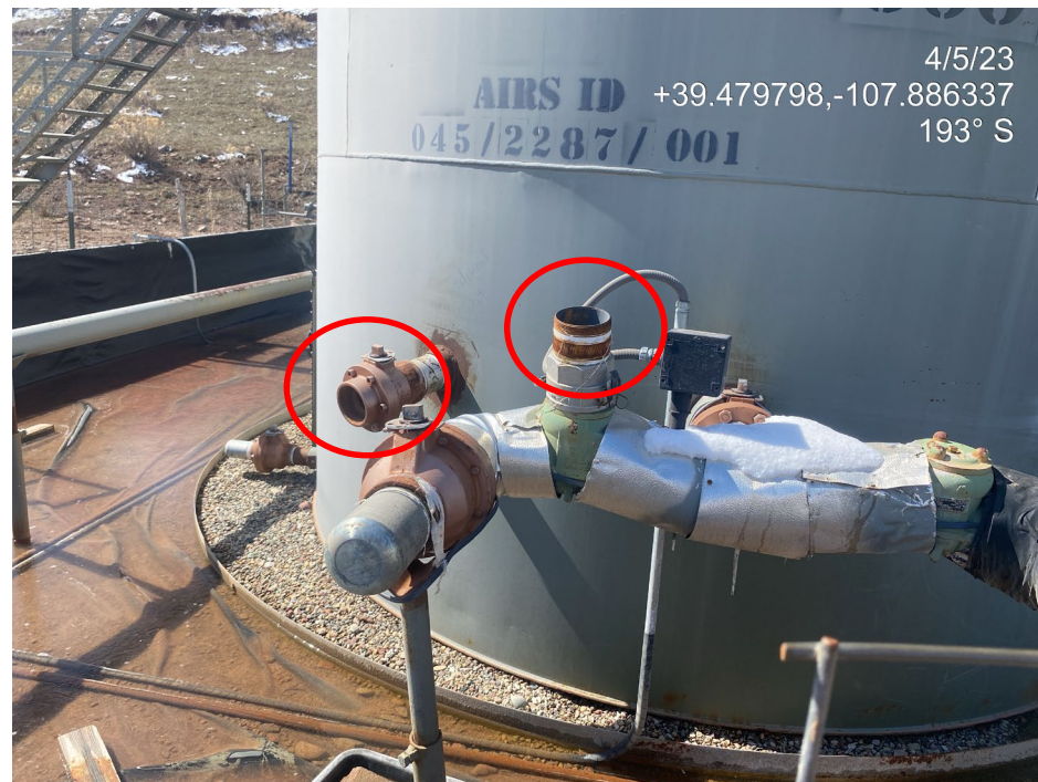
Photo 5. Photo shows bull plugs not installed on a tank line.
