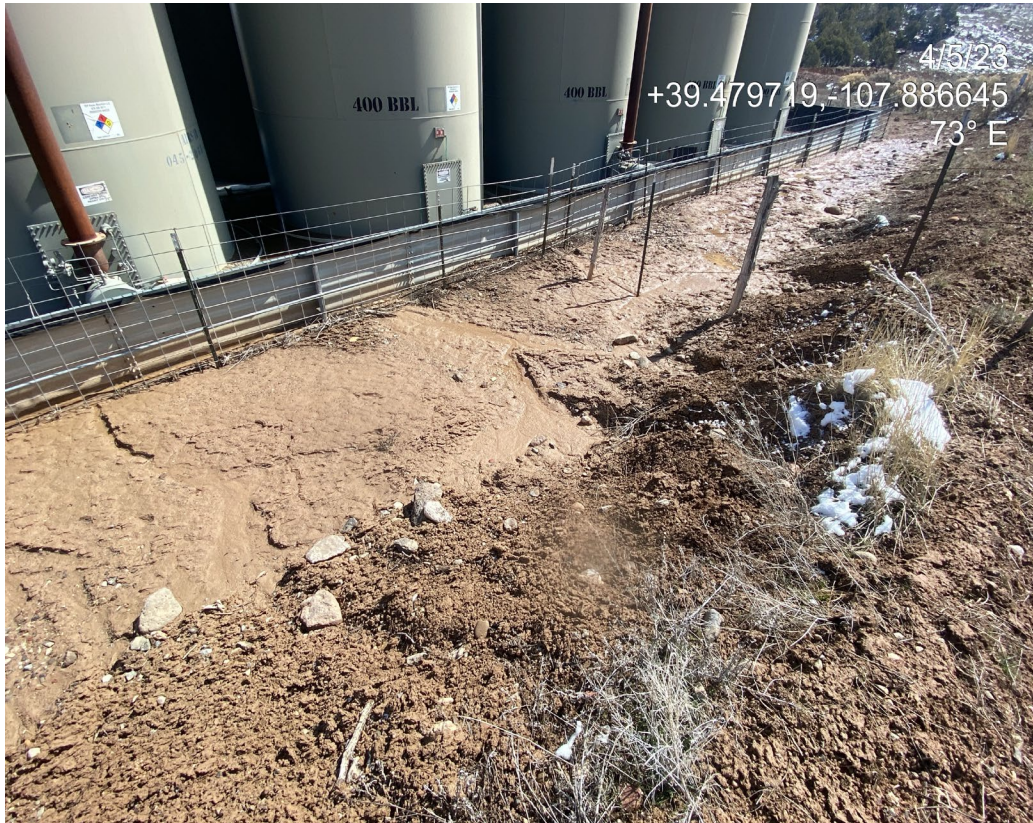
Photo 6. Photos show a berm at the south of the location is not stabilized. Rill erosion and sediment transport are evident.
