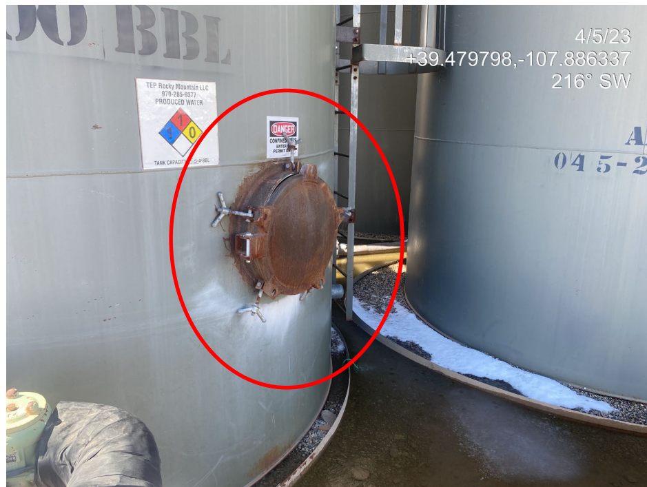
Photo 4. Photo shows a tank manway cover is not fastened and partially ajar.
