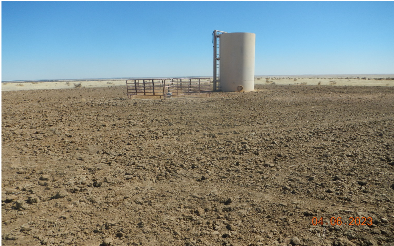
Photo 3. The compacted soils were ripped but unsure if cross-ripping was performed to 18inches. Disturbed soils will need to be seeded and stabilized.
