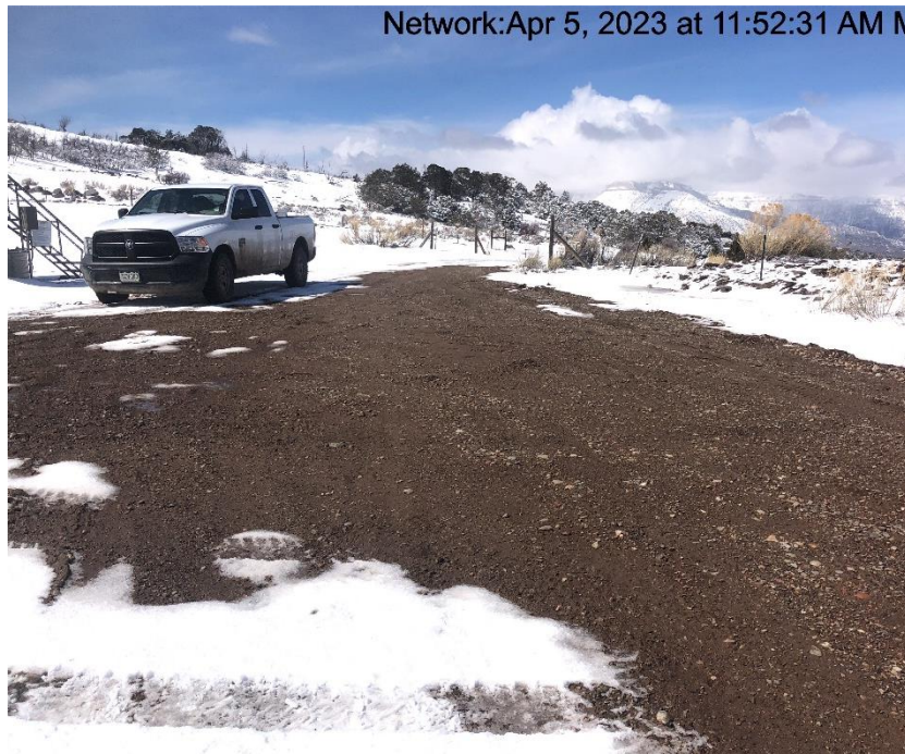
Photo #9551 insufficient tracking BMP at entrance to location
