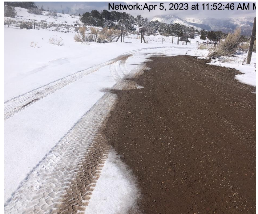
Photo #9552 insufficient tracking BMP at entrance to location
