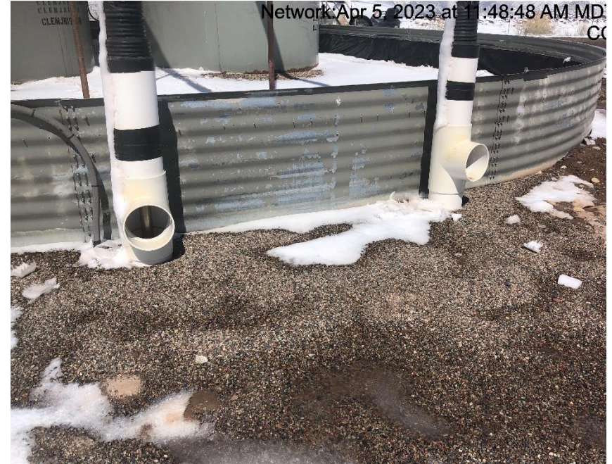
Photo #9541 Multiple places with flowline heating insulation open ended.
