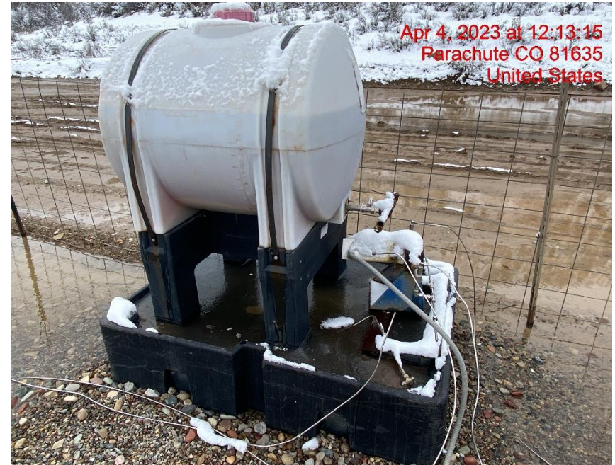
Inadequate Chemical Tank Secondary Containment Capacity – Photo #01895
