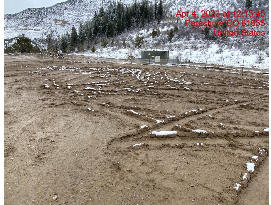
Lack of Stabilization w/ Inadequate Tracking BMP – Photo #01901
