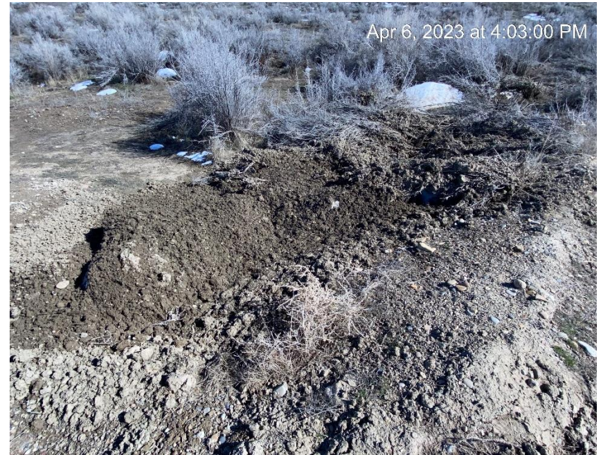
Sediment movement during snow removal
