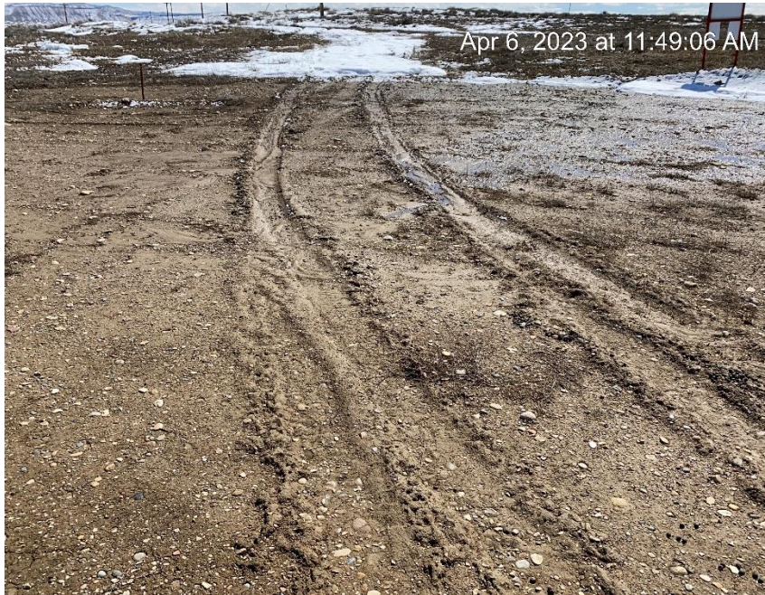
Traffic causing rutting and sediment migration
