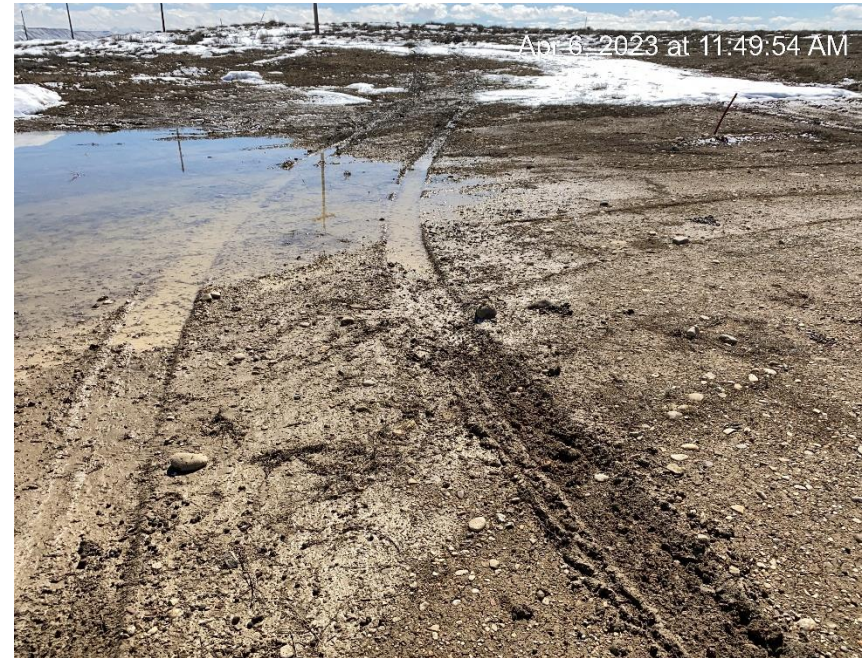
Lack of stabilization and vehicle tracking
