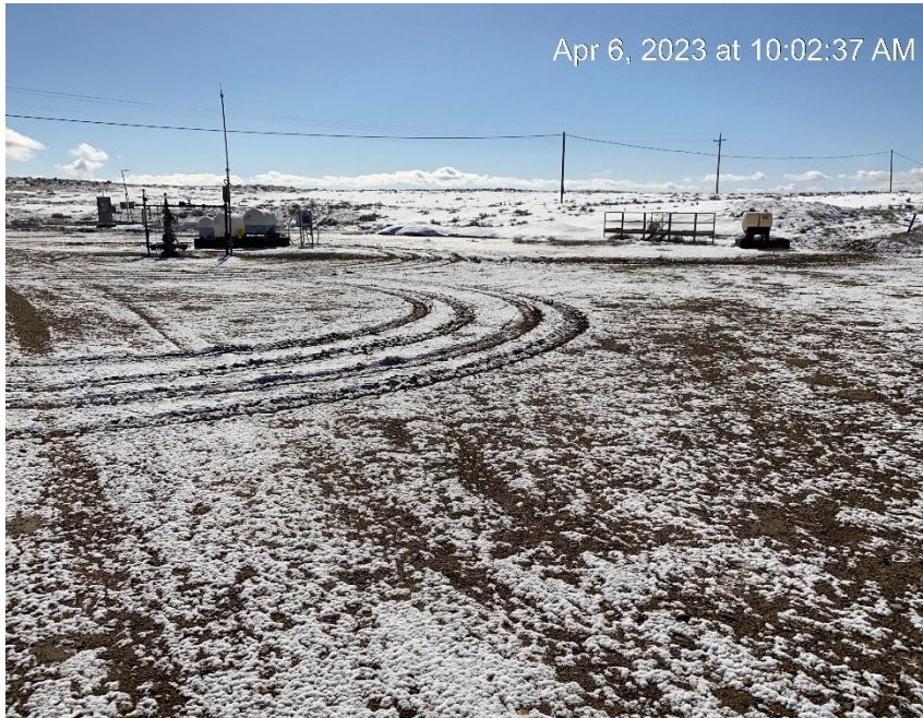
West location entrance
