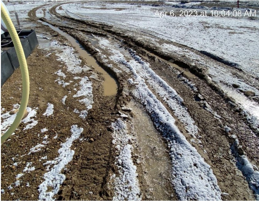
Lack of stabilization
