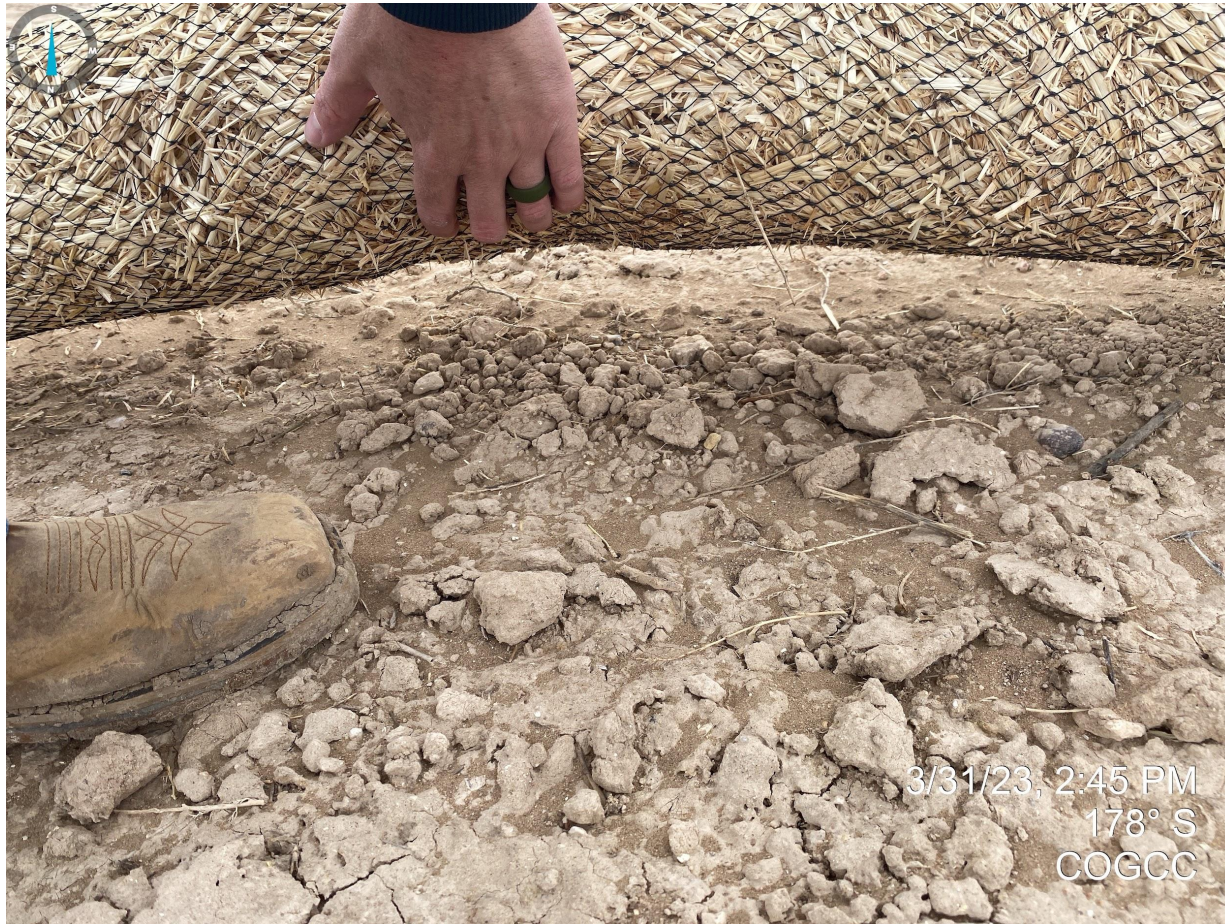
Photo 5. It does not appear the straw wattles were installed per good engineering practices as they were not trenched in. Sheet flow of water could potentially run directly underneath the straw wattles if not installed properly.
