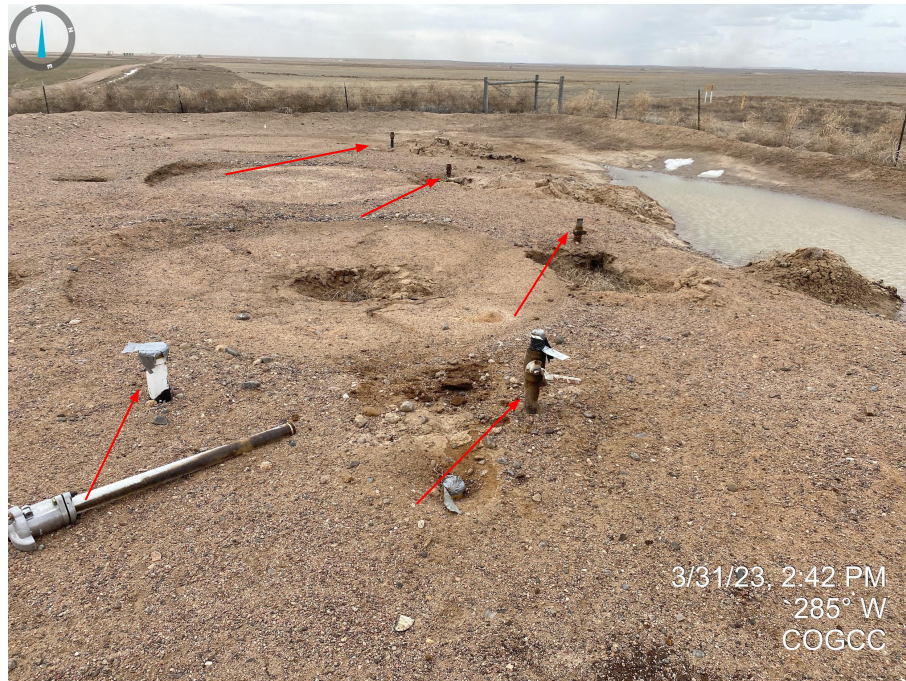
Photos 1 & 2. Abandoned risers do not have plugs or OOSLAT installed.
