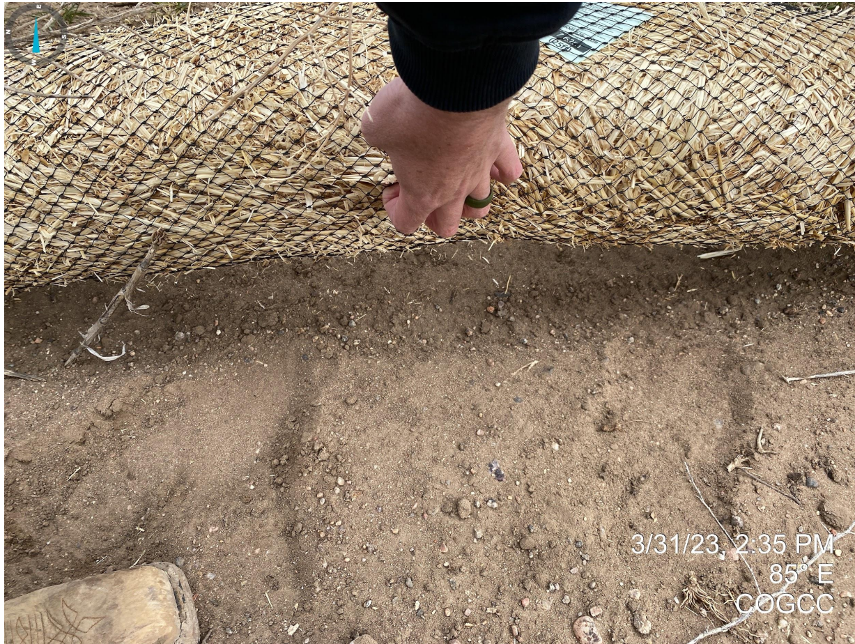
Photo 3. Close up photo illustrating that the straw wattles have not been trenched in per good engineering practices.
