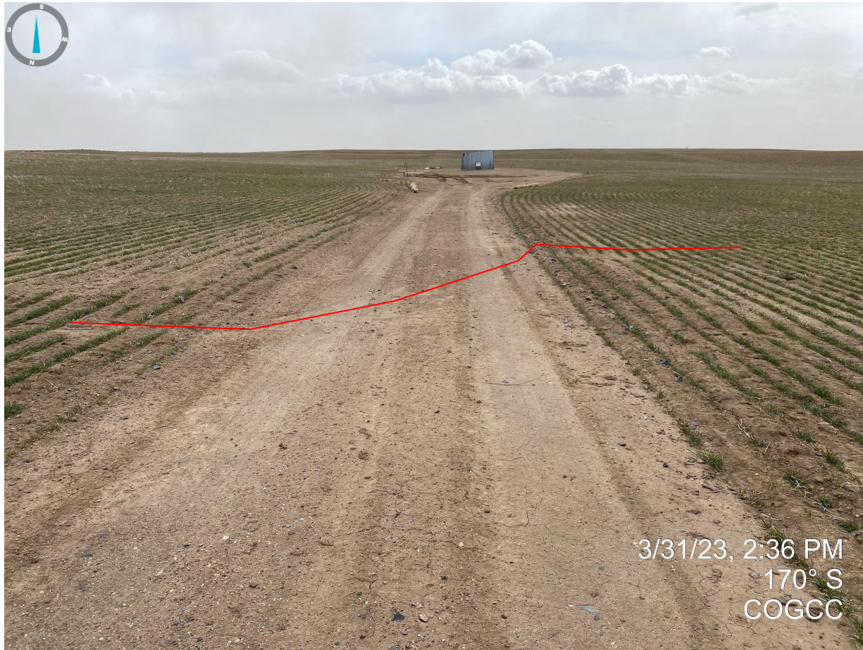
Photo 6. Overview illustrating rill erosion and path of stormwater. This area will need additional stormwater BMPs to prevent further erosion and degradation to adjacent lands.
