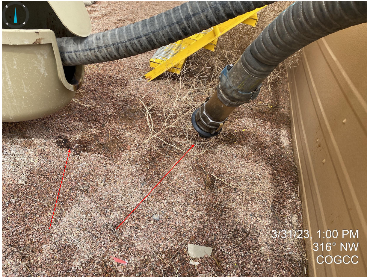
Photo 15. Oily waste observed on northeast side of tank battery.
