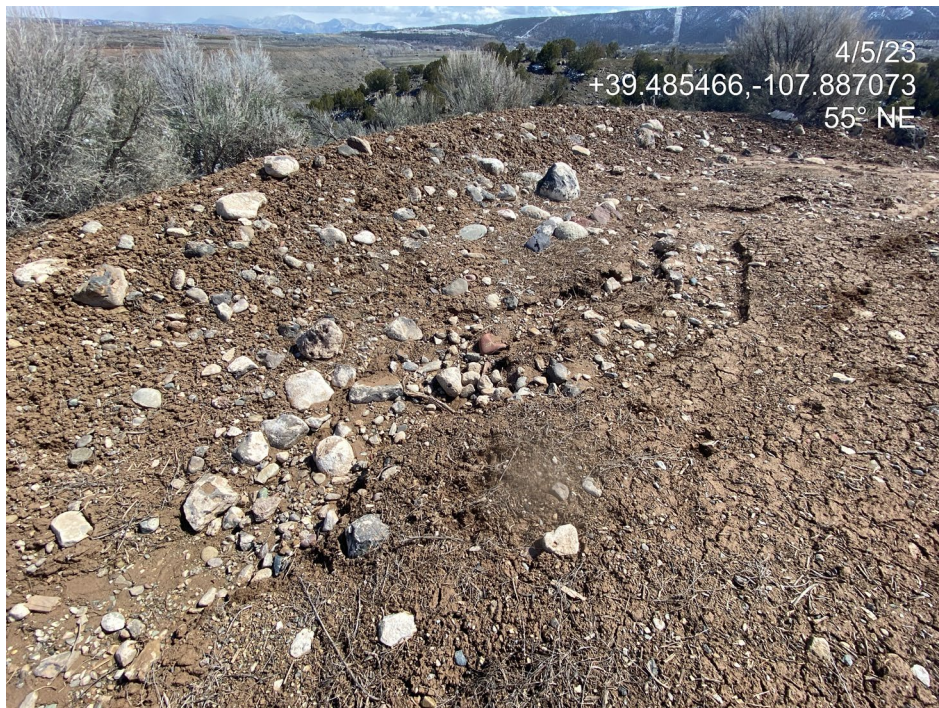
Photo 7. Photos taken from the north show lack of stabilization of the working pad surface (rill erosion). Photos show where stormwater flows into a plastic drain pipe (arrow) and what appears to be a small sediment trap (circled).
