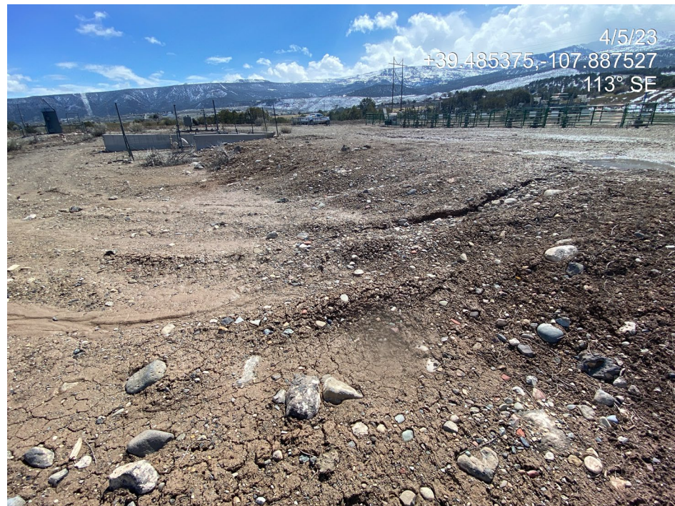
Photo 6. Photos taken from the north show lack of stabilization of the working pad surface (rill erosion).
