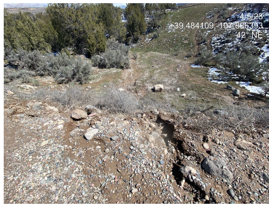
Photo 13. Photos show lack of stabilization of the access road (rills). Note the amount of road material (fine sediment and gravel) entering into the drainage.
