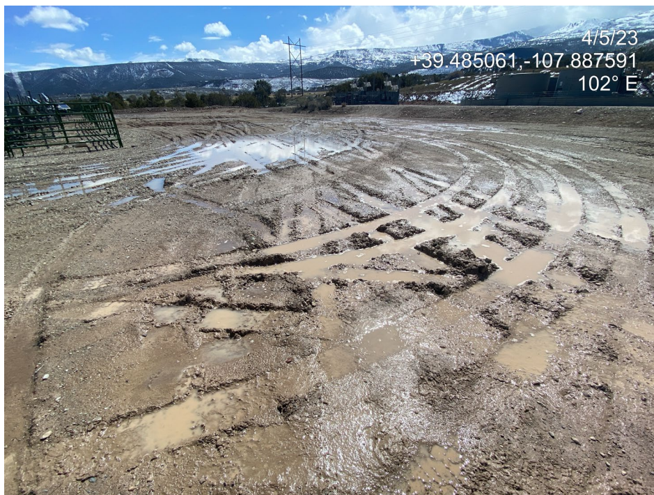
Photo 5. Photos show lack of stabilization of the working pad surface (ruts).
