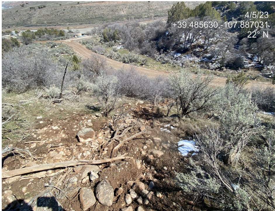
Photo 10. Photos taken just downslope of Photo 9 shows concentrated flows from the drain pipe resulting in rill erosion, sediment transport and offsite degradation.
