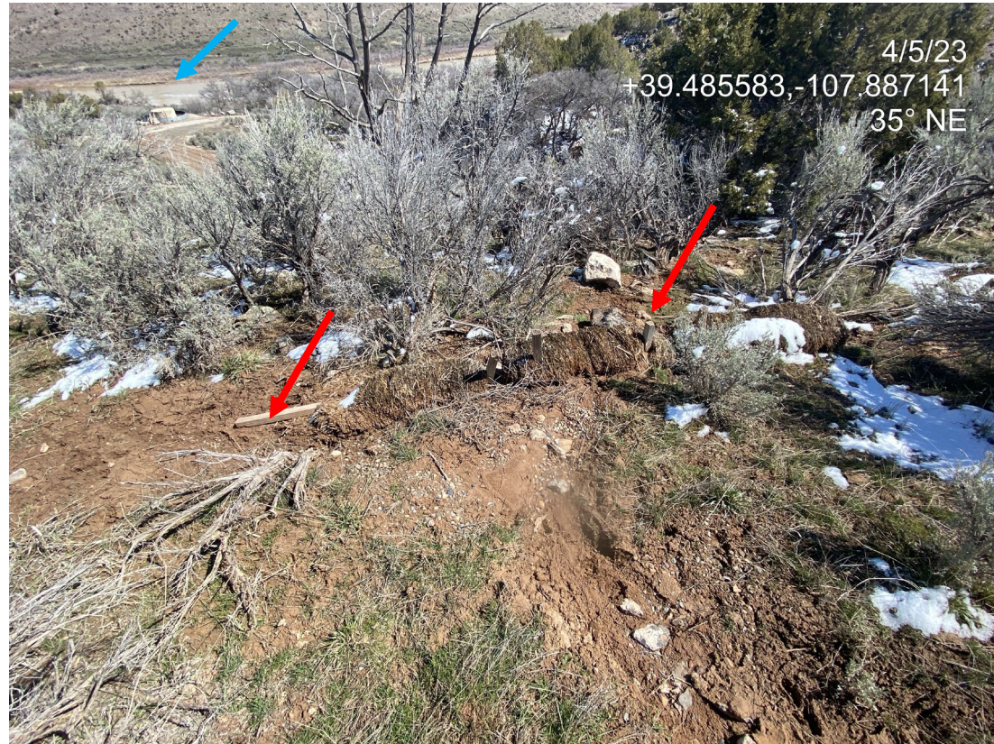
Photo 9. Photo taken just downslope of Photo 8 shows concentrated flows from the drain pipe resulting in rill erosion, sediment transport and offsite degradation. Sediment laden stormwater is bypassing straw bale BMPs (arrows). Note proximity to river (blue arrow).
