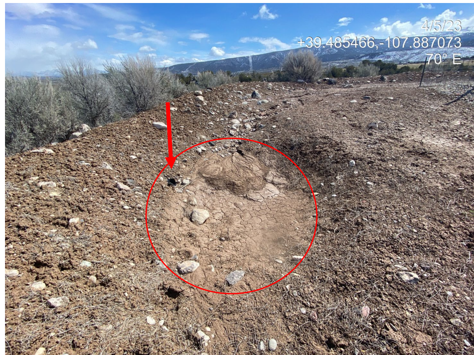
Photo 7. Photos taken from the north show lack of stabilization of the working pad surface (rill erosion). Photos show where stormwater flows into a plastic drain pipe (arrow) and what appears to be a small sediment trap (circled).
