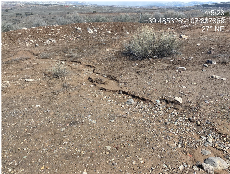
Photo 6. Photos taken from the north show lack of stabilization of the working pad surface (rill erosion).
