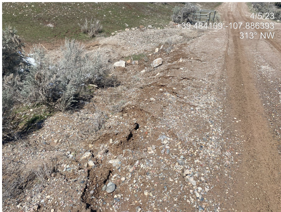
Photo 13. Photos show lack of stabilization of the access road (rills). Note the amount of road material (fine sediment and gravel) entering into the drainage.
