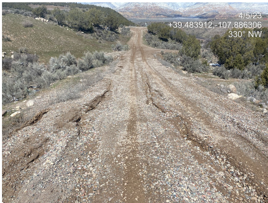
Photo 12. Photos show lack of stabilization of the access road (rills).
