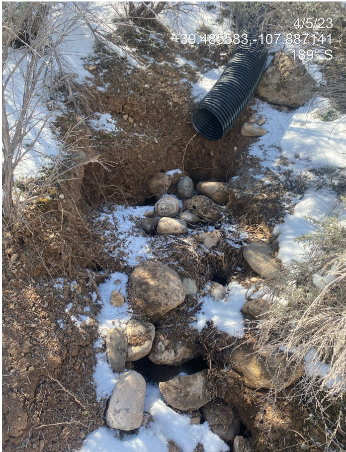
Photo 8. Photo shows the outlet for the drain pipe shown in the previous slide (left). Outlet protections are degraded, insufficient and resulting in degradation.
