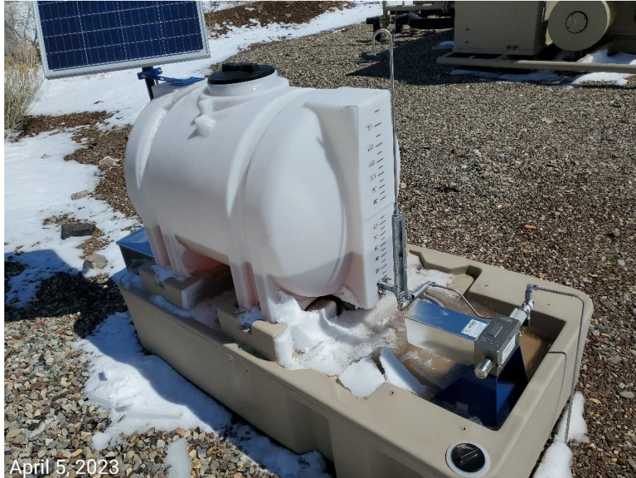
Photo 2: Chemical container lacks required marking/labeling/signage.
