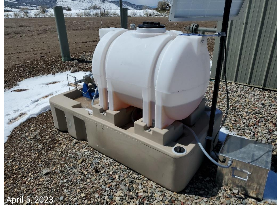
Photo 2: Chemical container lacks required marking/labeling/signage.
