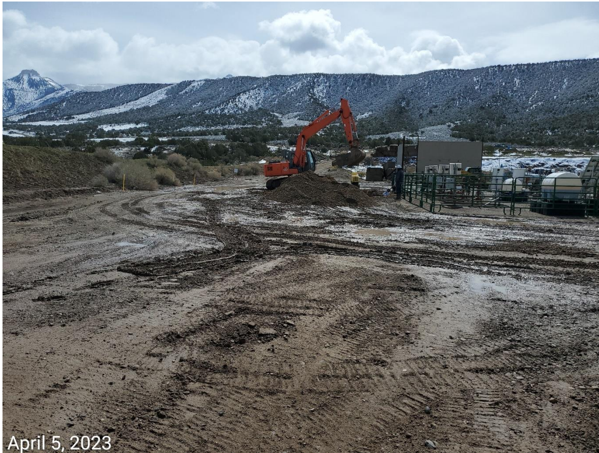
Photo 11: Backfilling excavation in process. BMPs at excavated soils not observed.
