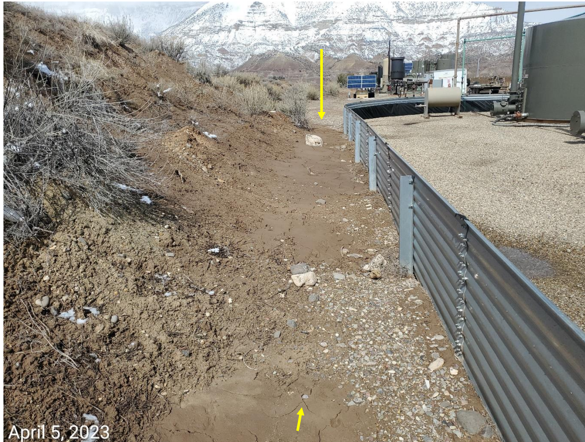
Photo 5: Photo shows sediment deposition due to unstabilized cut slopes.
