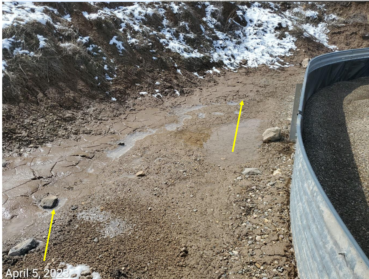
Photo 4: Photo shows sediment deposition due to unstabilized cut slopes.
