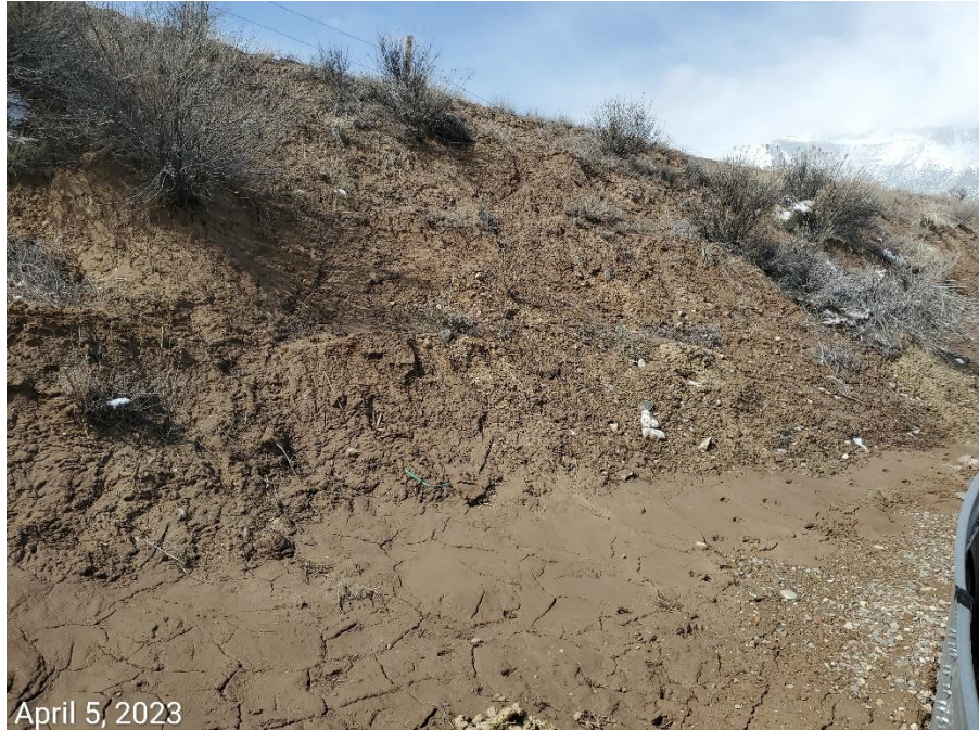
Photo 3: Photos taken from the cut slopes on the southwest end of the Location. Photos show slopes lack stabilization- erosion degradation evident.
