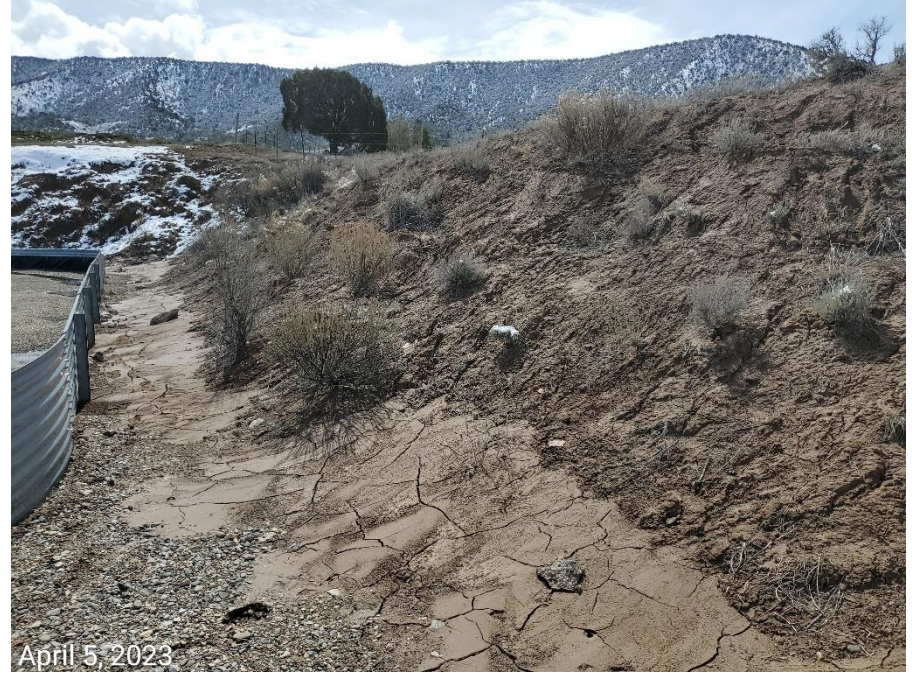
Photo 3: Photos taken from the cut slopes on the southwest end of the Location. Photos show slopes lack stabilization- erosion degradation evident.
