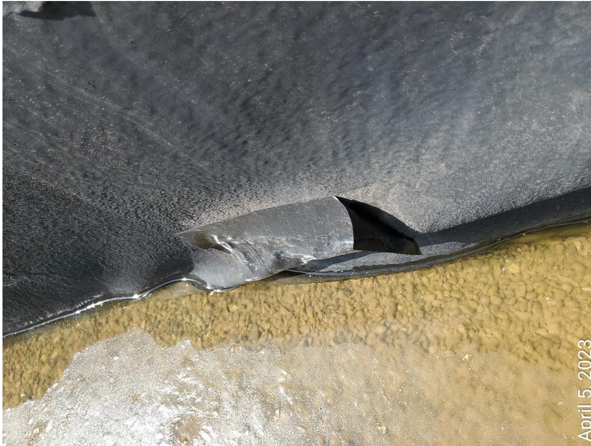
Photo 2: Repair work to liner inadequate- patch is peeling off.
