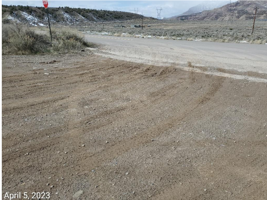
Photo 6: Photos show sediment transport from access road onto public roadway has continued.
