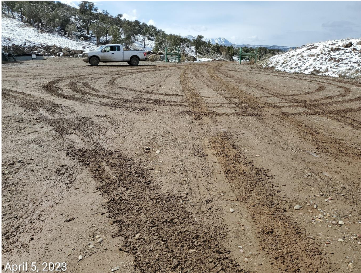
Photo 5: Tracking BMPs showing signs of disrepair.
