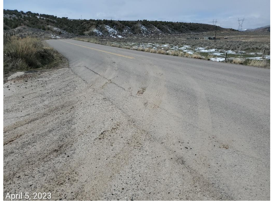
Photo 6: Photos show sediment transport from access road onto public roadway has continued.
