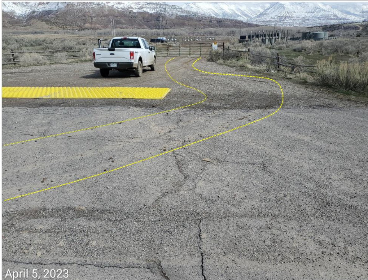
Photo 1: Photos 1-3 taken from the access road entrance and Stone Quarry Road. Photo shows Operator has implemented a single row of “reusable trackout control mats”. BMP is not per good engineering practices, and is inadequate in length to allow for at least an entire tire rotation for most off-highway, or industrial vehicle tires used in O&G. Photo also shows that Operator is traveling around the VTC (yellow dotted lines), resulting in continued sediment transport onto the public roadway.
