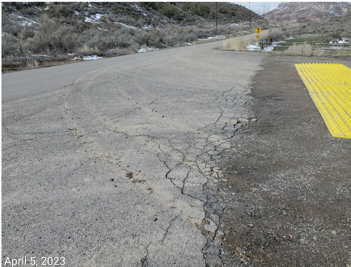
Photo 2: See comments under photo 1. Photo shows sediment transport from the Location onto the public roadway has persisted.
