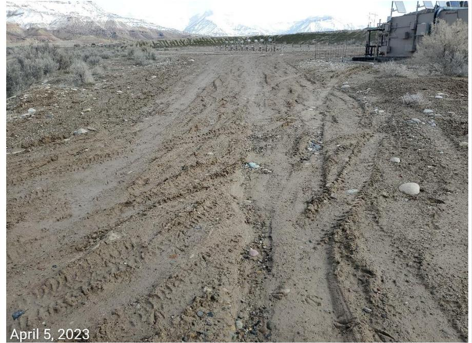
**Photo 1:** Photos 1-3 taken from the Location. Photos show BMPs to stabilization the Location, and to minimize erosion, degradation and off-site sediment transport remain missing or insufficient.
