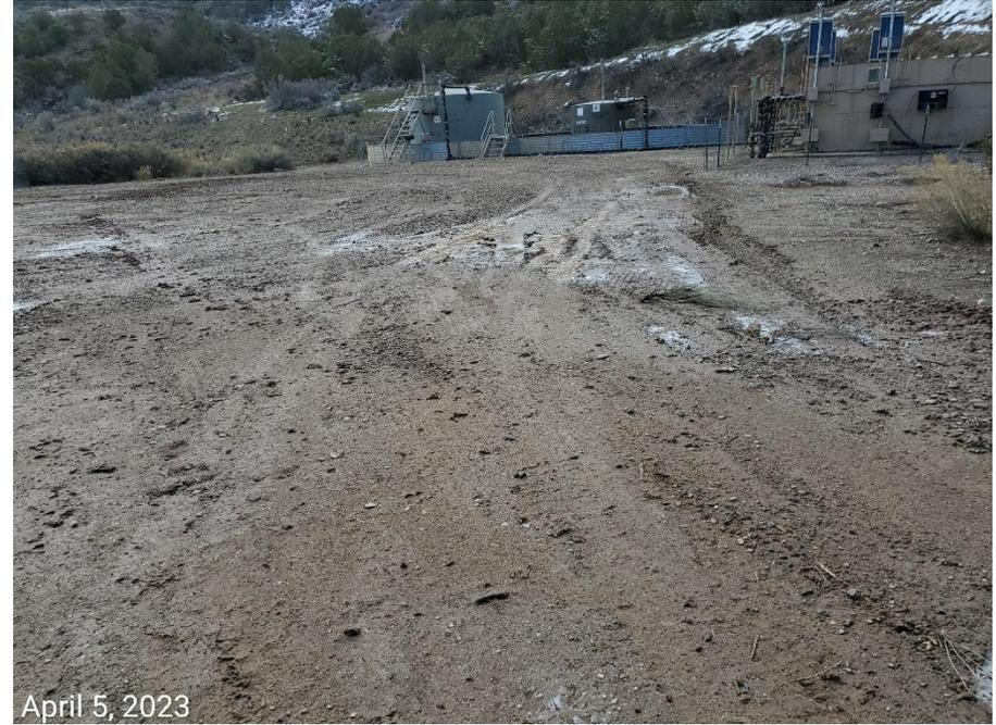
**Photo 1:** Photos taken from the Location entrance. Photo shows Operator appears to have re-graded the working pad- regrading alone is inadequate to provide long-term stabilization, minimization of degradation, tracking and off-site sediment transport, and is considered a temporary repair measure.
