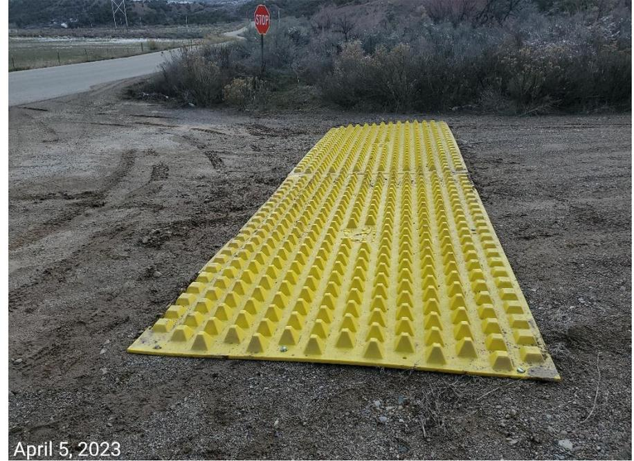
**Photo 2:** Photo taken from the access road entrance. Photo shows Operator has implemented a single row of “reusable trackout control mats”. BMP is not per good engineering practices, and is inadequate in length to allow for at least an entire tire rotation for most off-highway, or industrial vehicle tires used in O&G.
