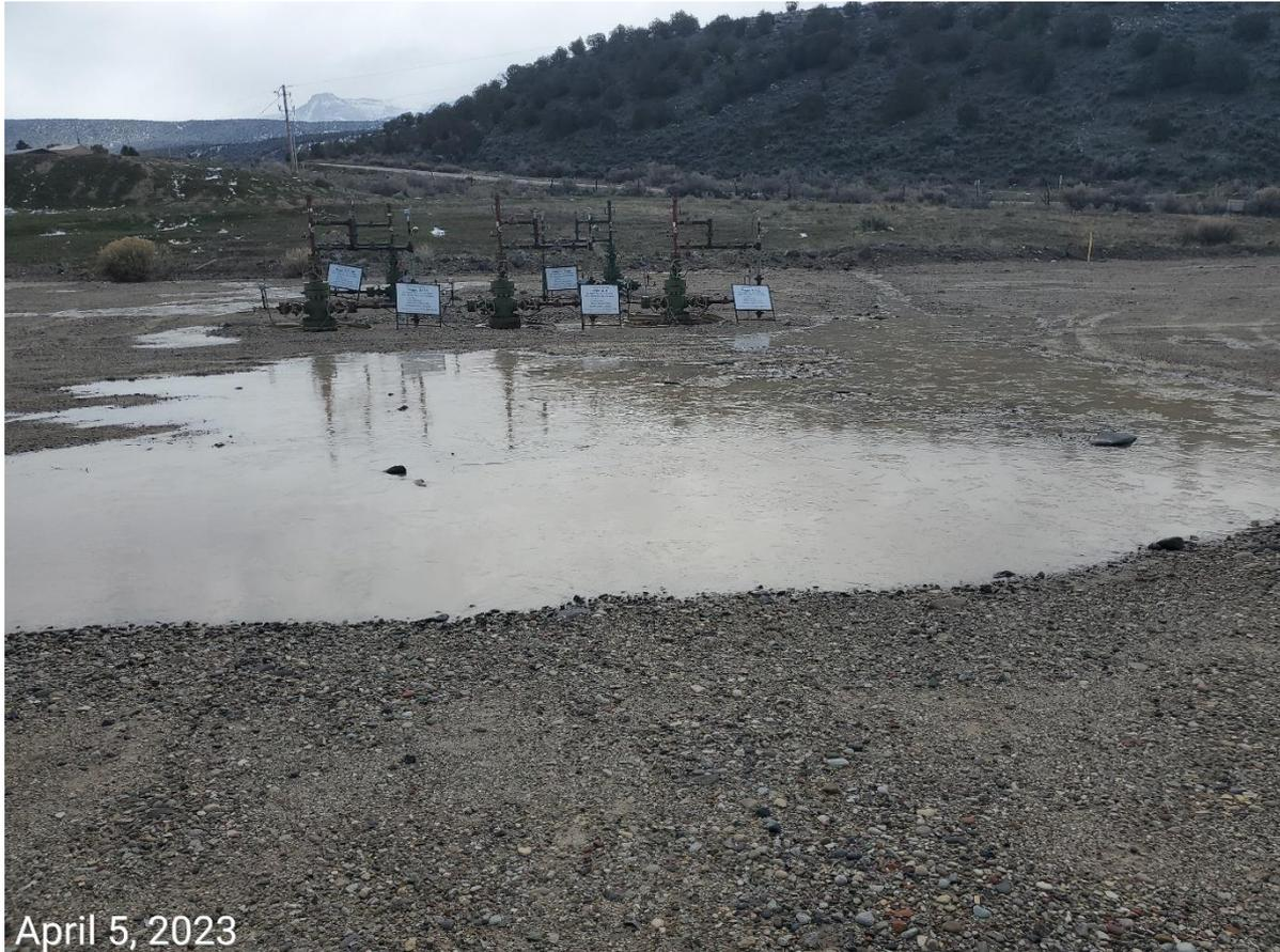
**Photo 3:** Photo shows stormwater ponding on the Location. BMPs inadequate to allow for proper stormwater discharge. Photo shows conditions/BMPs appear to remain unchanged since prior inspections, and appear to discharge runoff onto the working pad, rather than from.
