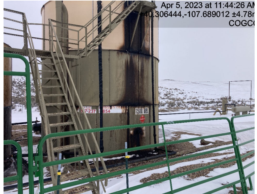
Possible leaks on tank or was over filled
