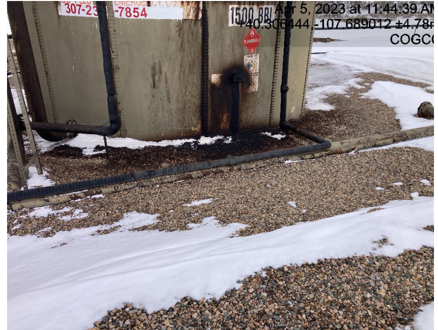
Staining and possible leak on tank
