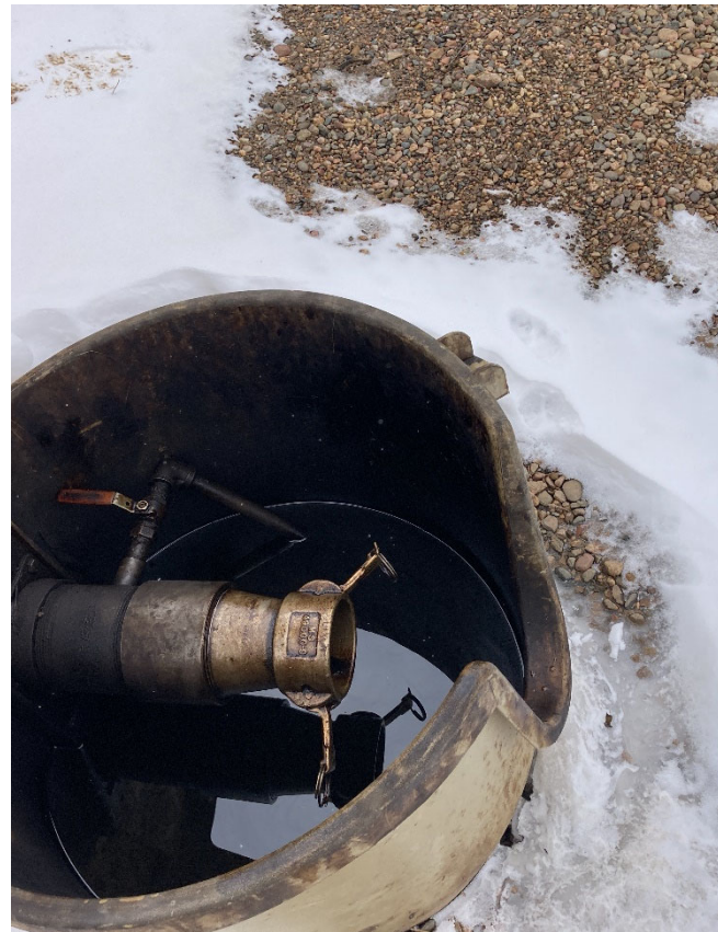
Valves on tanks missing caps/plugs
