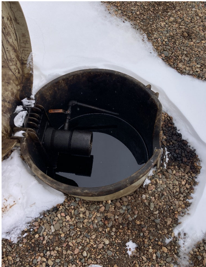
Valves on tanks missing caps/plugs
