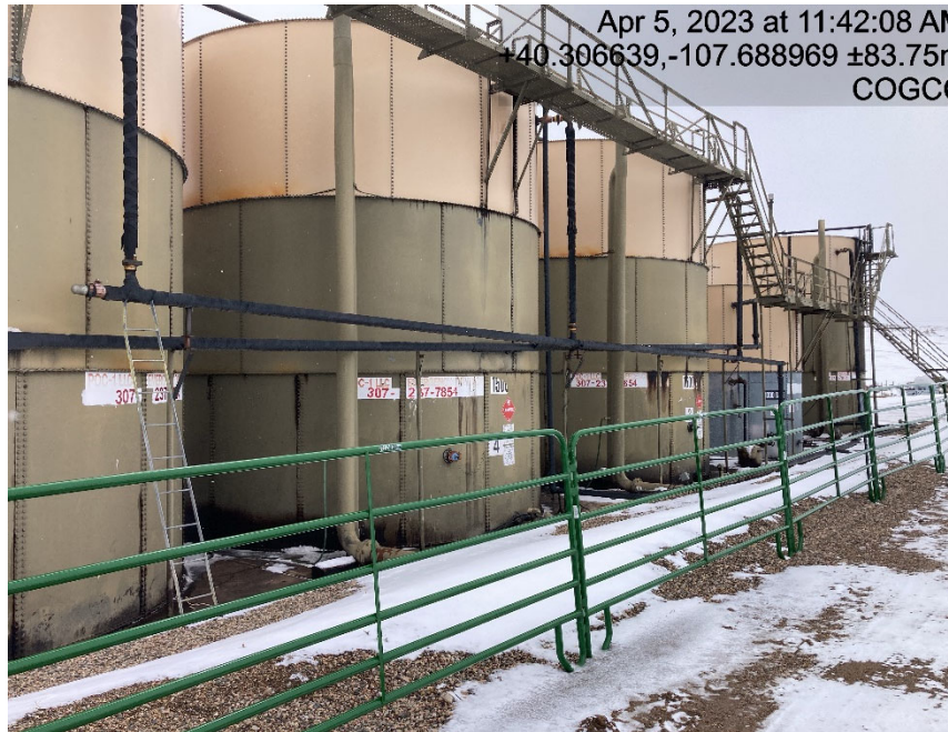
Location and lack of proper battery signage
