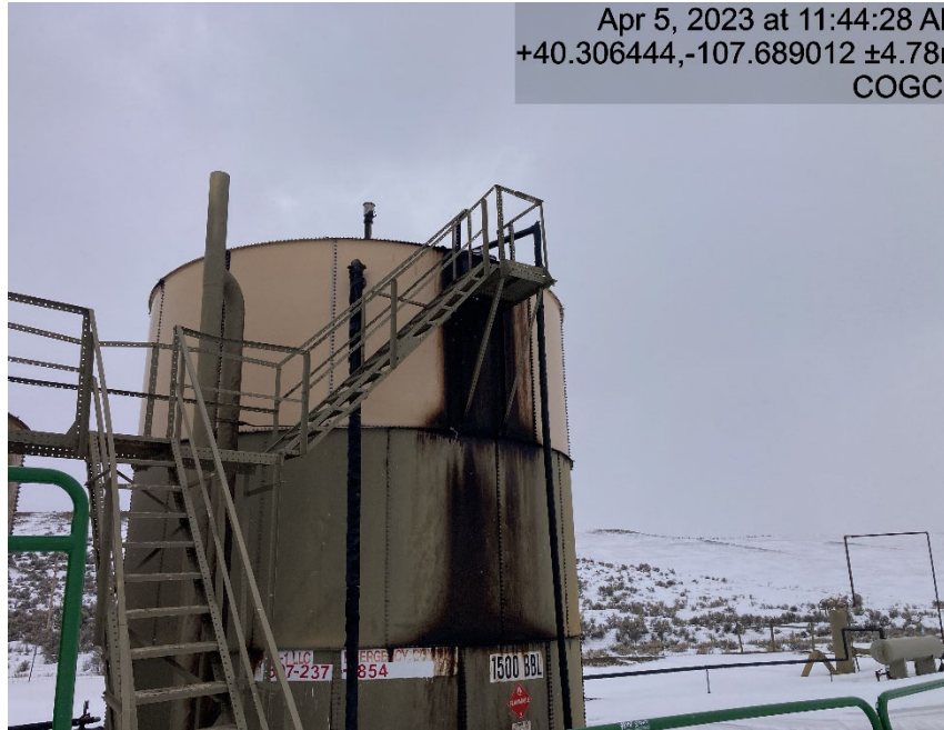
Possible leaks on tank or was over filled
