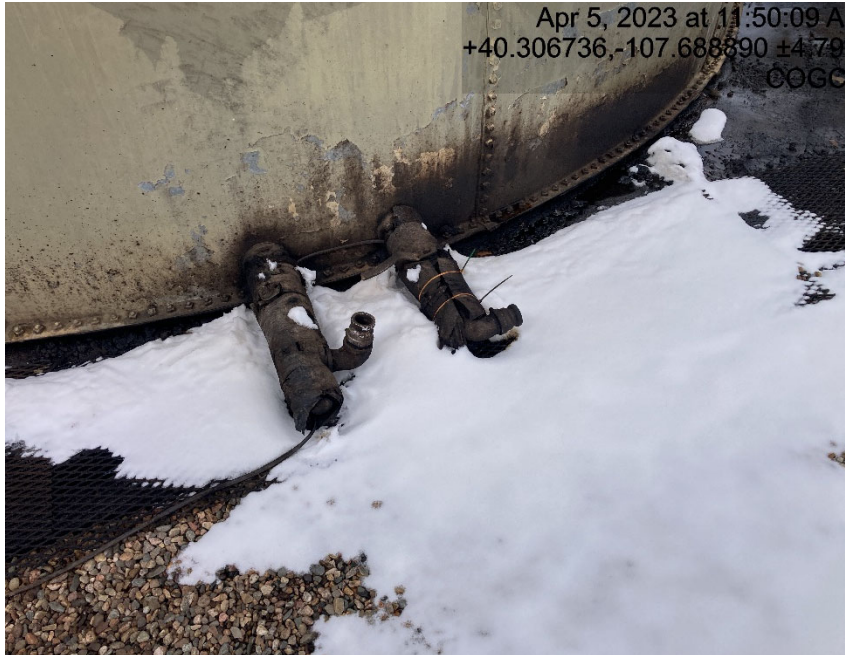
Valves on tanks missing caps/plugs
