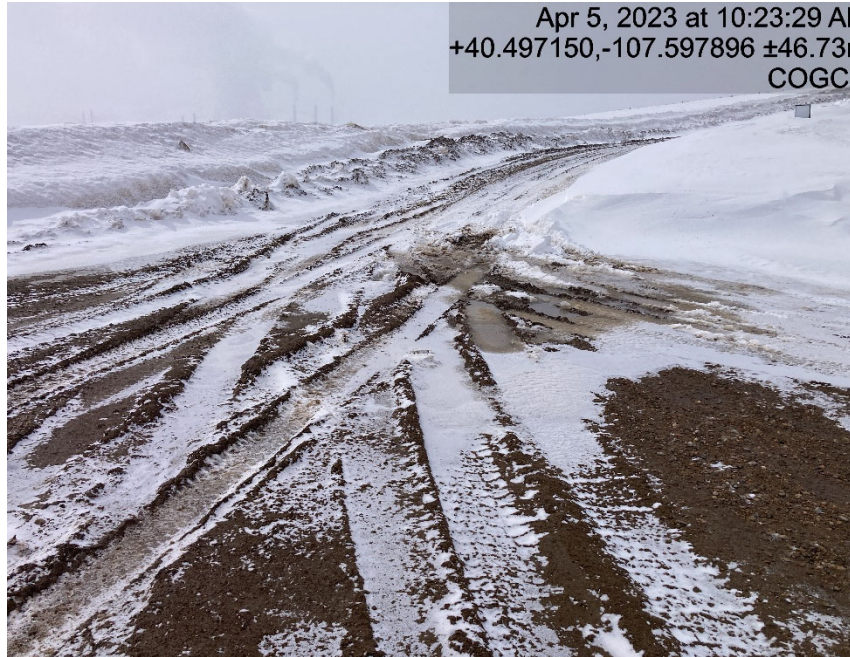
Location entrance show signs of lack of stabilization and lacking tracking BMP's
