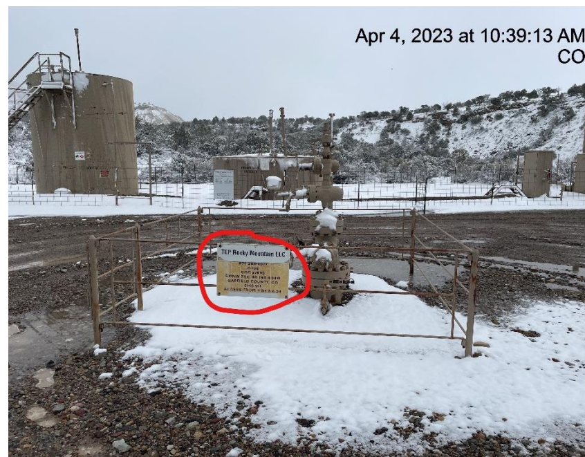
Photo # 4222 Wellhead sign missing required information
