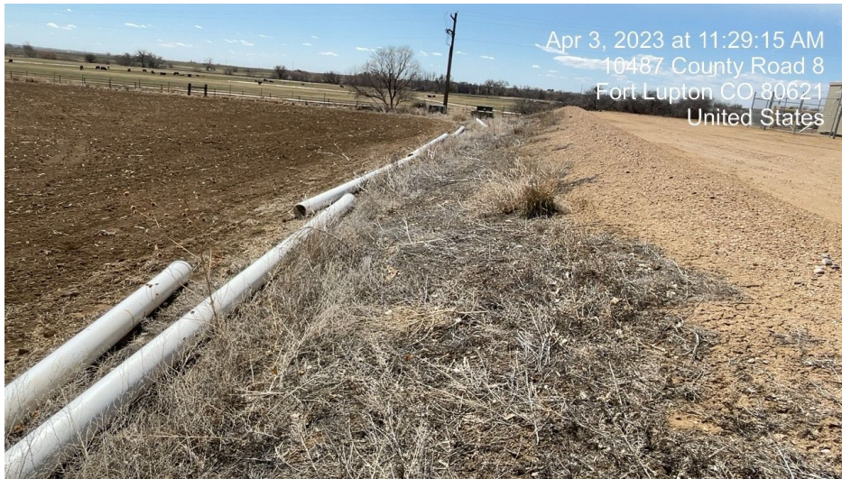
Photo 3. Photo taken of weeds and debris on fill slope of production pad
