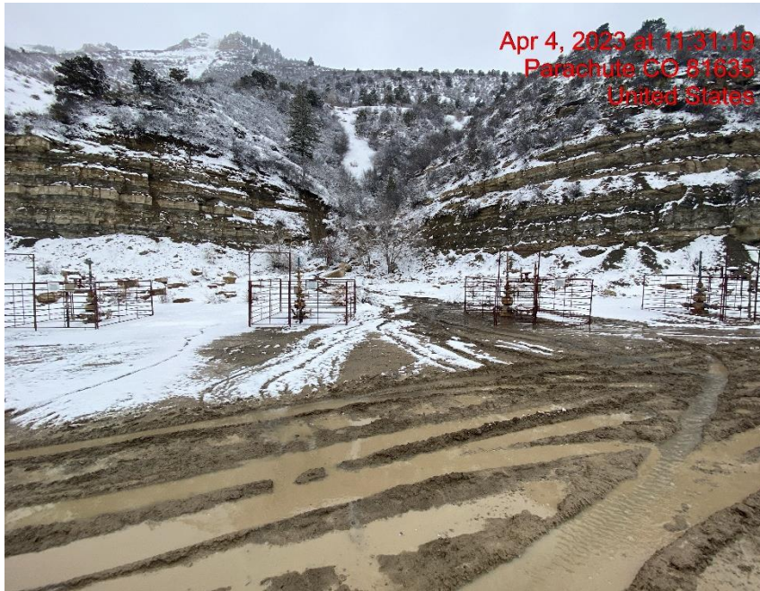
Wellheads/Lack of Stabilization – Photo #01870
