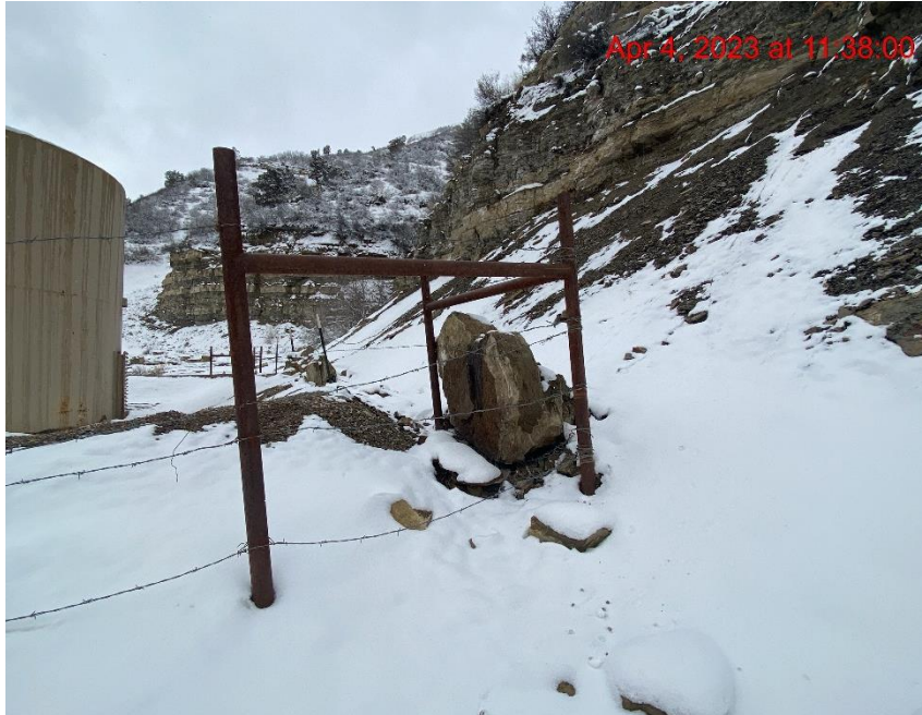
Cut Slope Erosion/Run-On – Photo #01877
