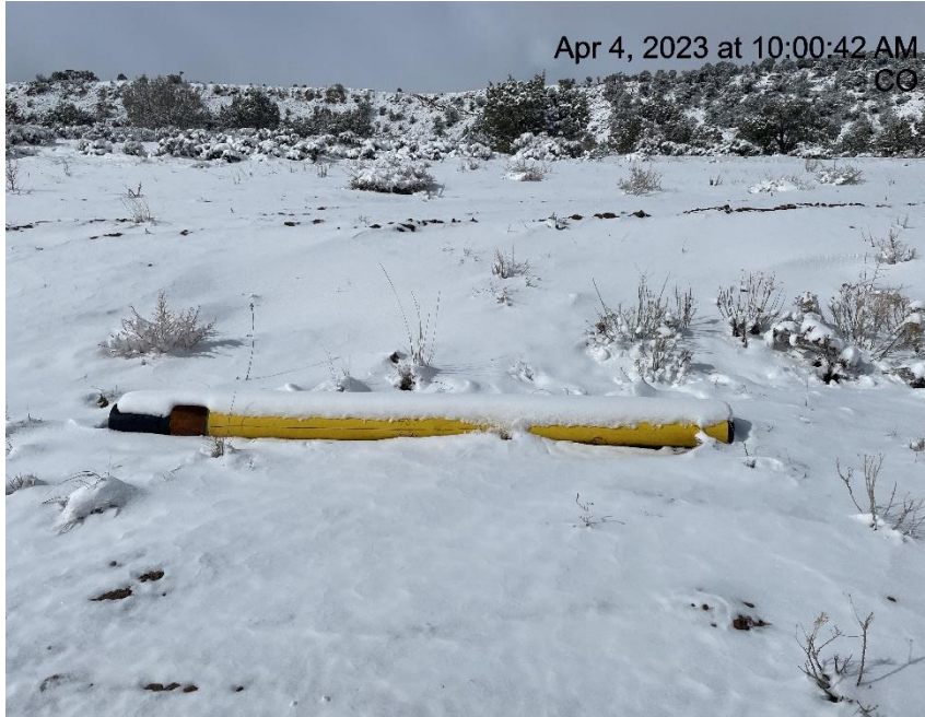
Photo # 4154 Debris along spur road
