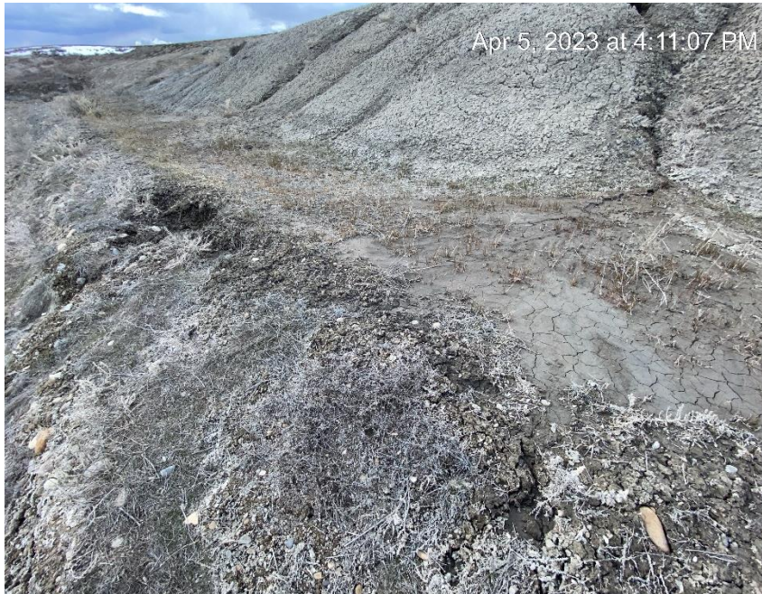
Diversion ditch full of sediment and erosion onto location
