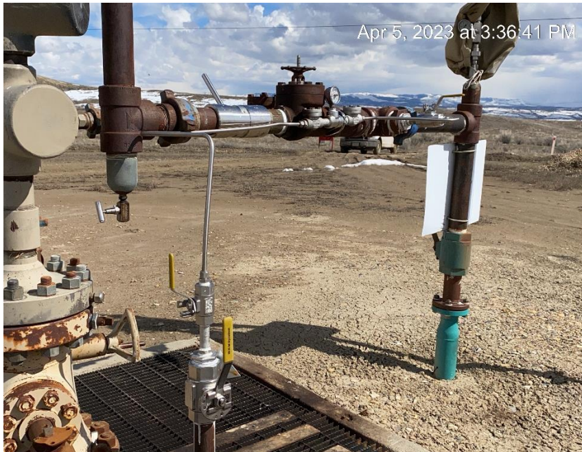
Bradenhead line connected to flowline
