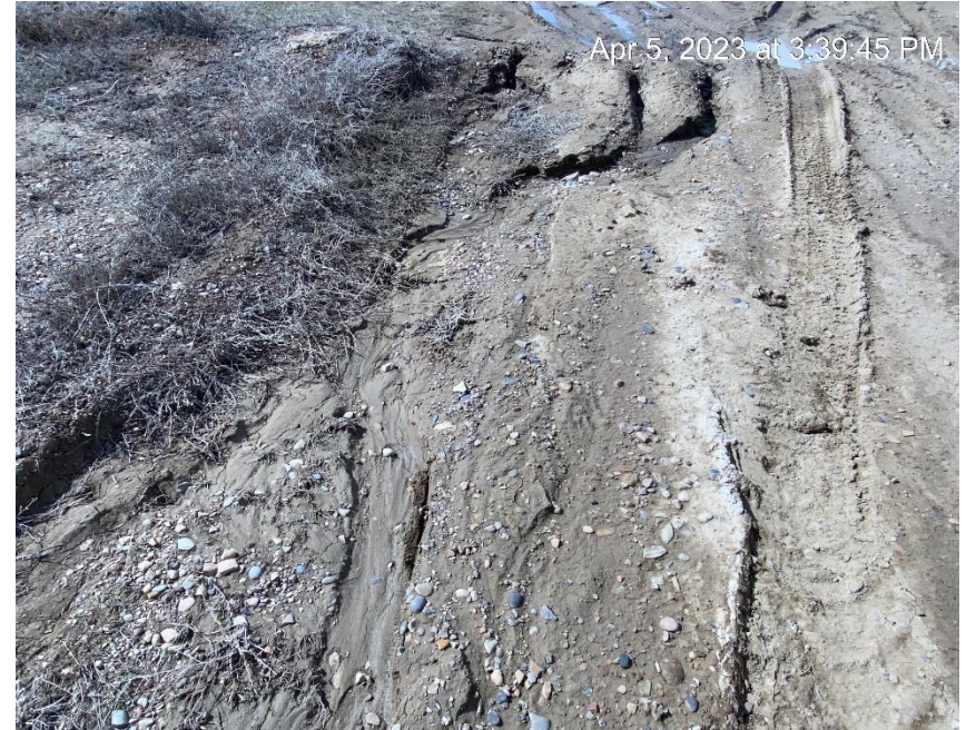
Location and lease road erosion and sediment migration
