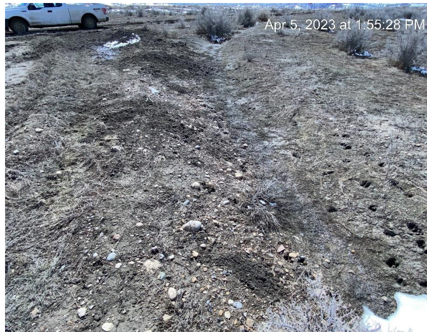
Soil pushed into drainage ditch during snow removal
