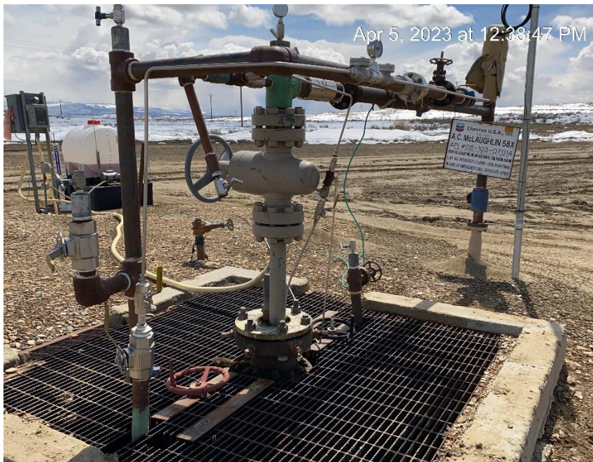
Wellhead. Line off Bradenhead to flowline.
