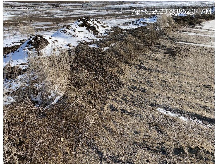
Sediment deposited outside location berm
