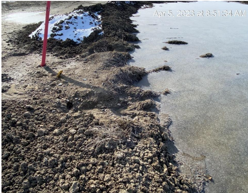
Breached location berm
