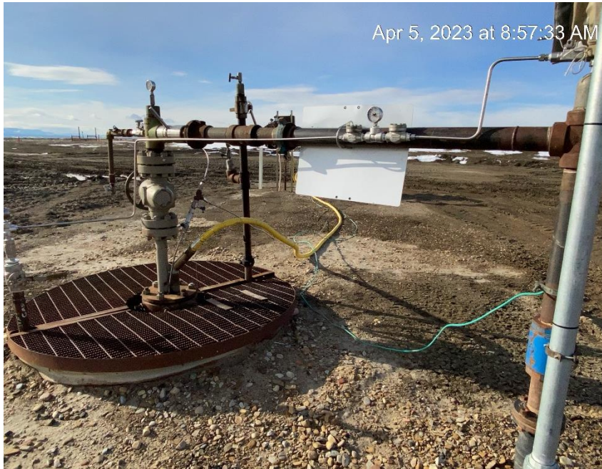
Bradenhead line to flowline
