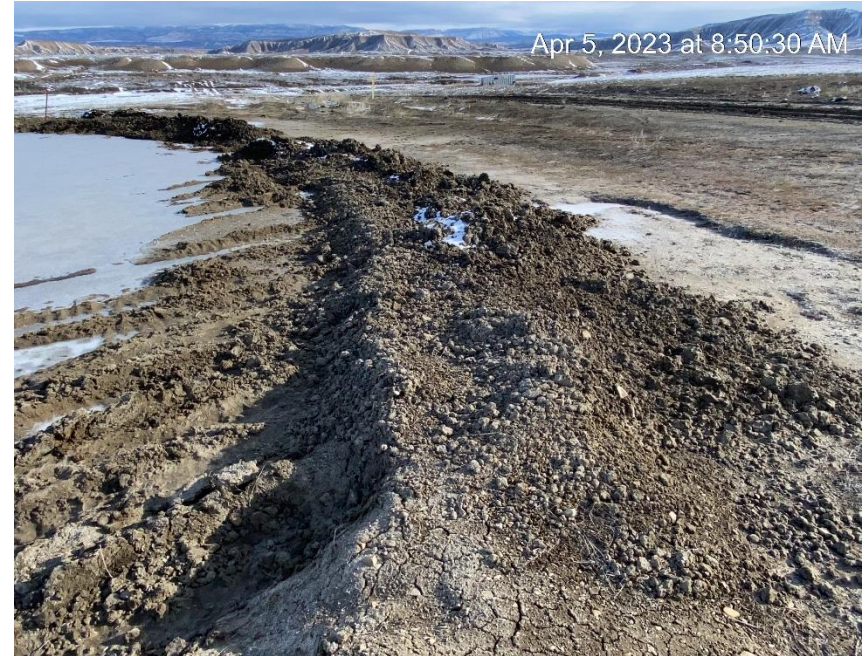
Sediment deposited outside location berm
