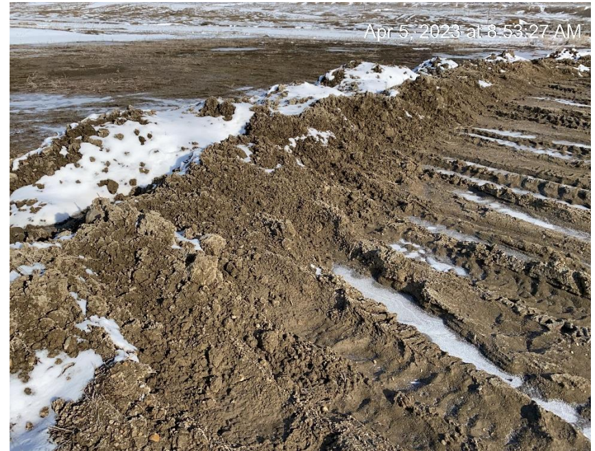
Sediment deposited outside location berm
