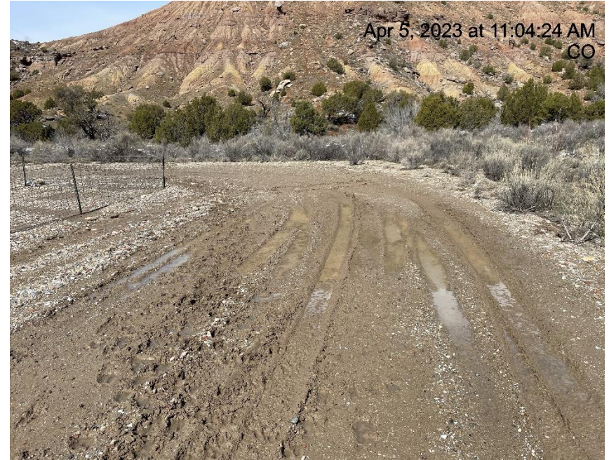
Photo # 4312 Lack of stabilization/insufficient tracking BMP's
