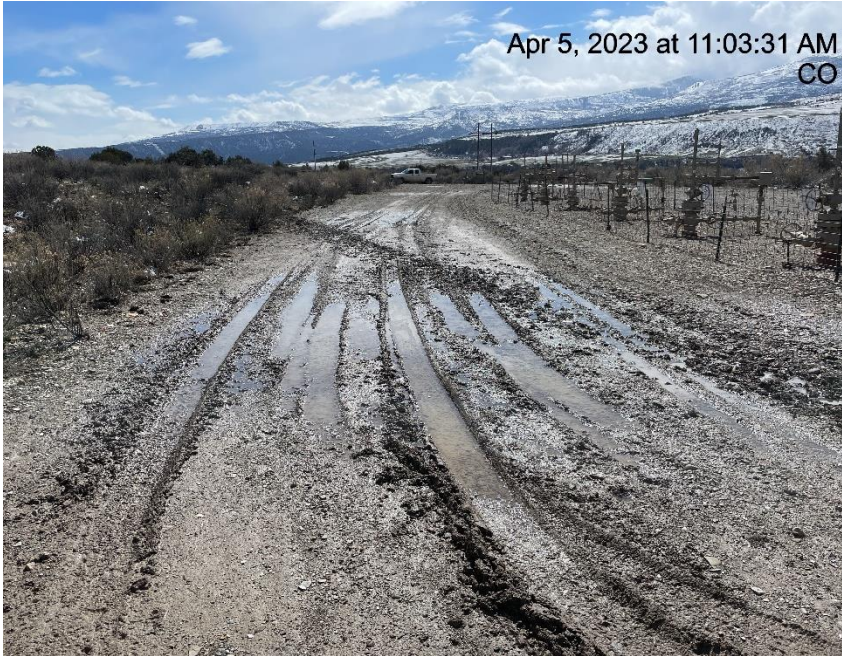
Photo # 4310 Lack of stabilization/insufficient tracking BMP's
