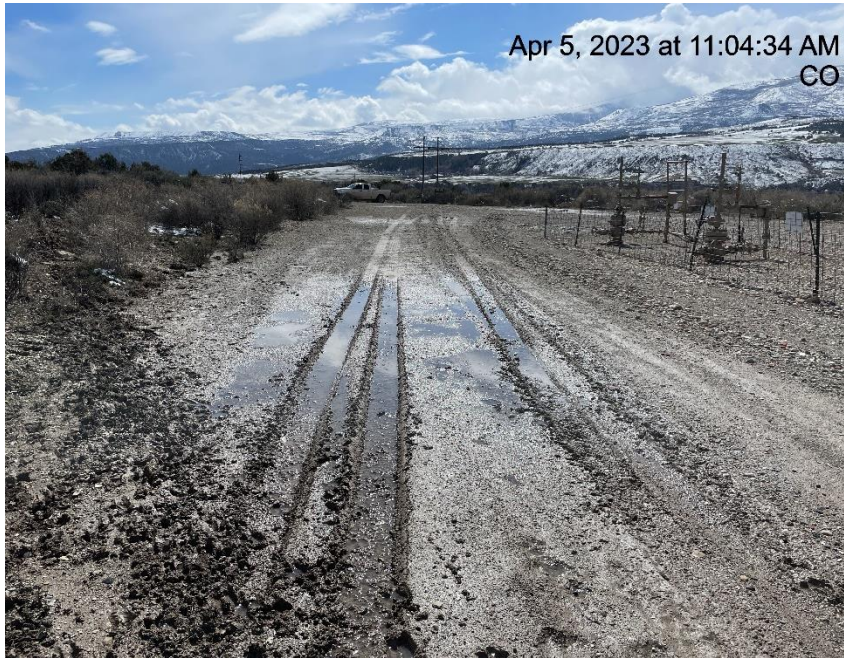
Photo # 4313 Lack of stabilization/insufficient tracking BMP's
