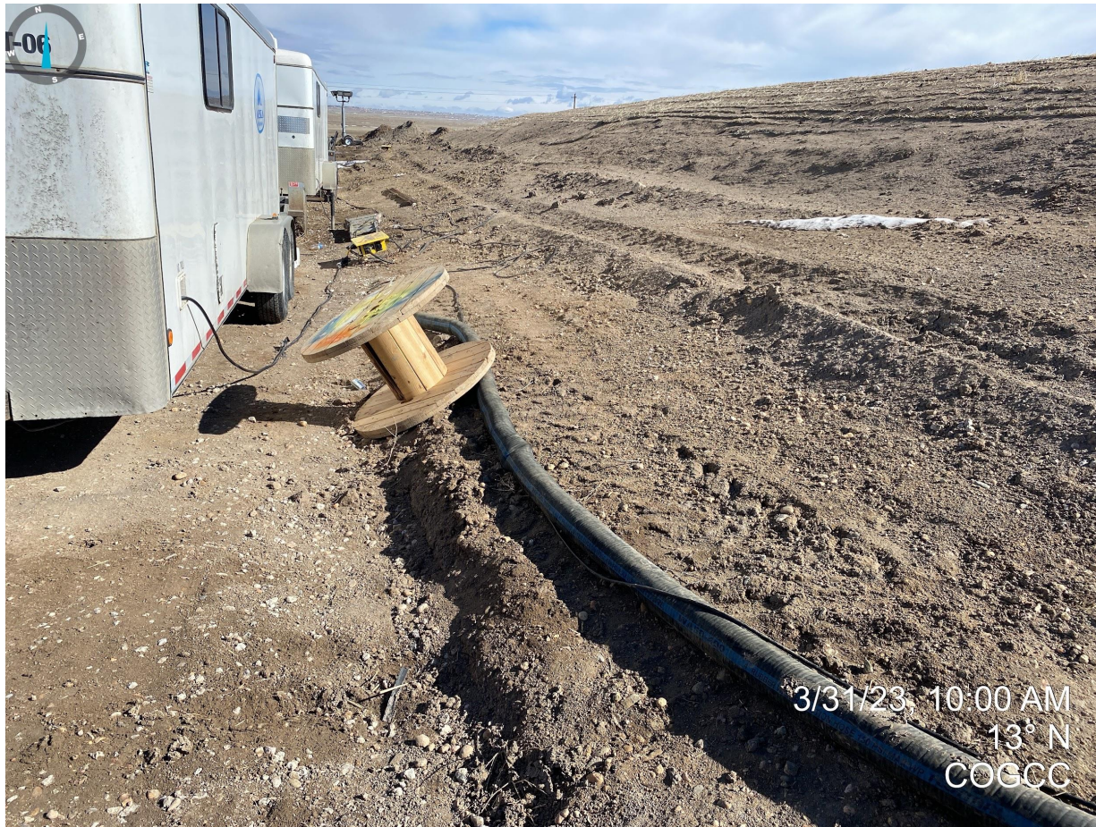
Photo 26. Facing north from the western portion of the topsoil stockpile. Photo illustrates equipment being stored on the stockpile, and the absence of stabilization BMPs on this portion of the stockpile.
