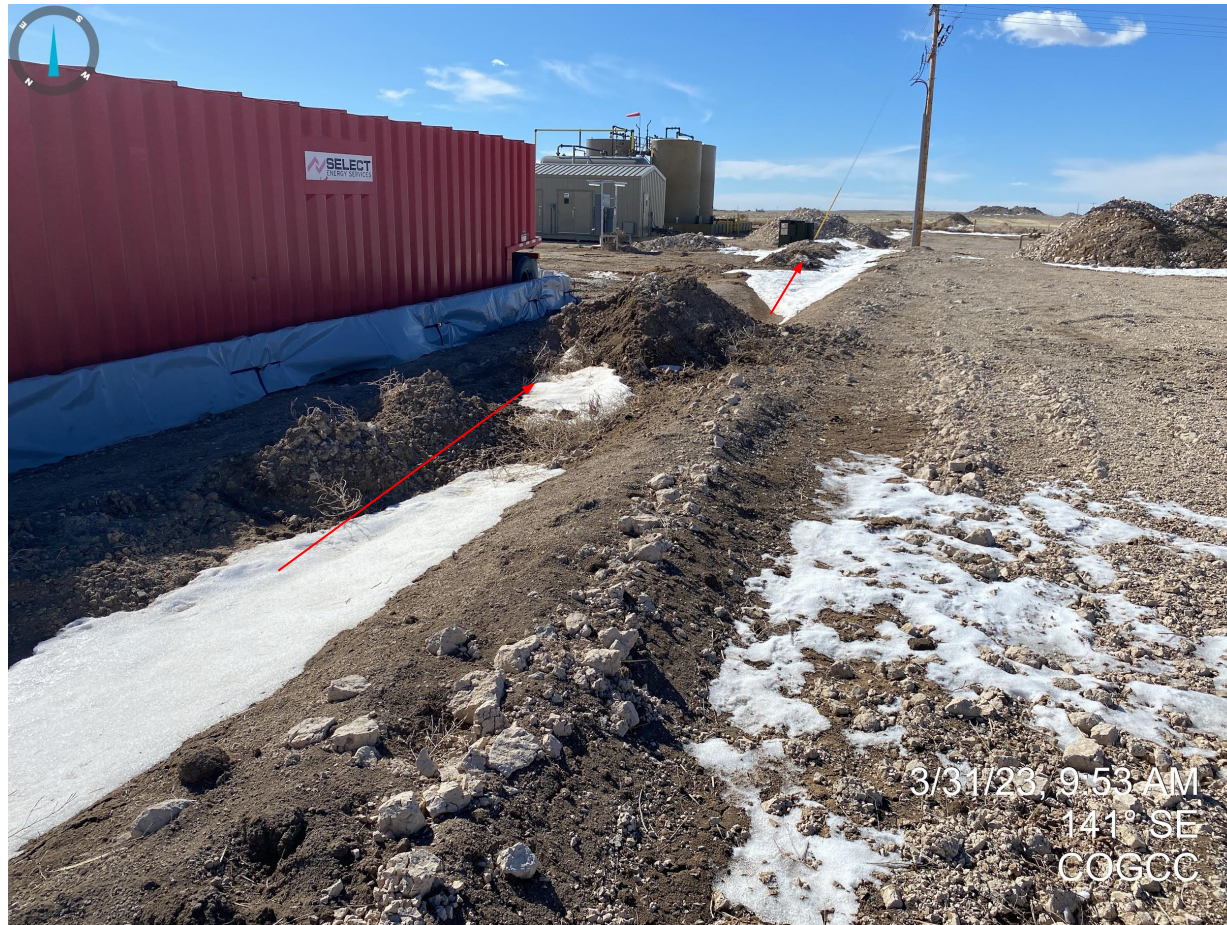
Photo 9. Facing southeast from central/western ditch and berm; material placed/stored within stormwater ditch.
