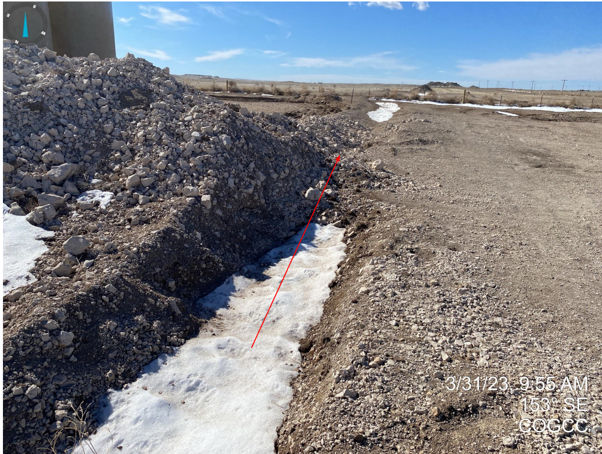
Photo 14. Facing south; material being stored in the stormwater ditch.
