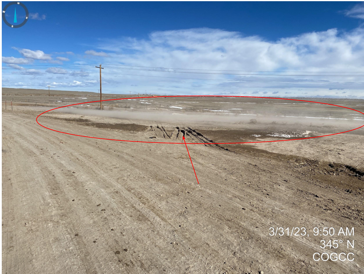
Photo 2. Facing north near the entrance to the pad. Photo illustrates that the location has not been properly stabilized with evidence of wind erosion and dust blowing off location. Additionally, vehicle tracks were observed going through the interim areas and not staying on the access/lease road (red arrow).
