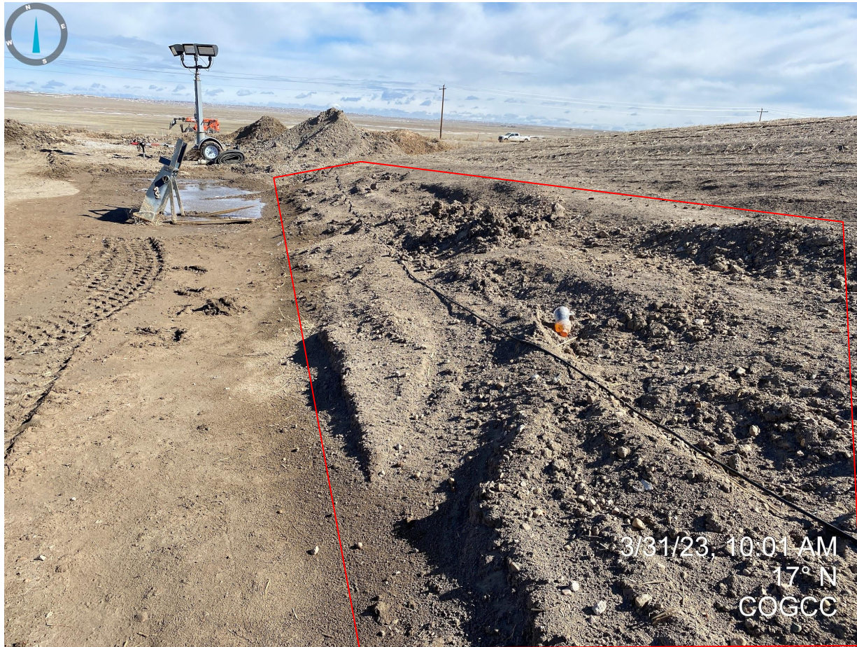
Photo 28. Facing north at the northern end of stockpile. Photo illustrates unconsolidated topsoil that is susceptible to wind and water erosion as it is not properly stabilized.
