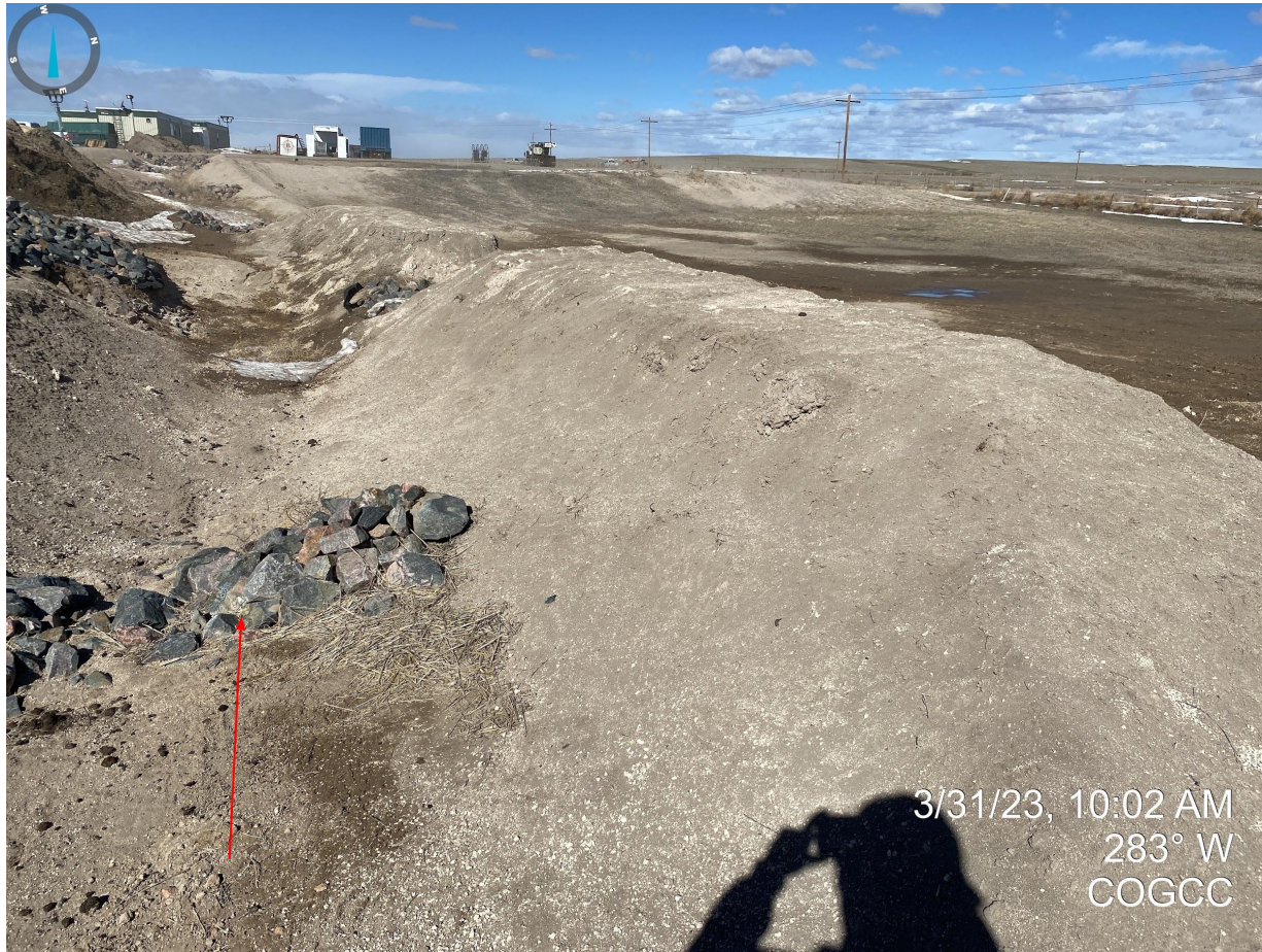
Photo 32. Facing west at northern portion of location. Berm BMPs does not appear to be an adequate BMP as the walls are nearly vertical, comprised of unconsolidated material (or lacking stabilization techniques), and have evidence of rill erosion (out of view). Additionally, rip rap check dams require maintenance as they are filled with sediment.
