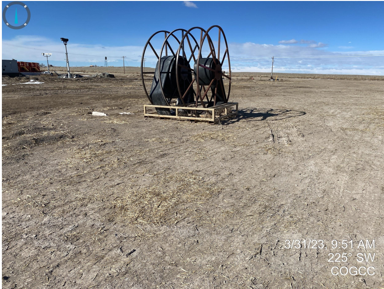
Photo 4. Facing southwest near the location entrance. Materials/supplies were being stored within the recently seeded/reclaimed area. Additionally, this reclaimed area is not properly stabilized as most of the straw mulch has blown away and Staff observed dust originating and blowing off location from this area.
