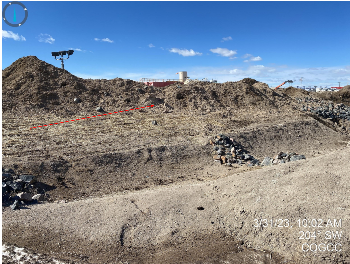
Photo 34. Facing southwest near sediment trap. Photo illustrates unconsolidated material placed next to stormwater ditch. The unconsolidated material can become a potential source of pollution itself as it is not properly stabilized.
