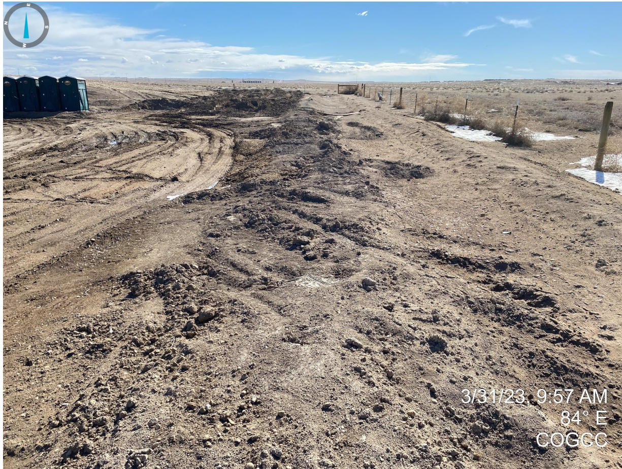
Photo 17. Facing east at southern portion of location. Photo illustrates that this portion of the ditch is comprised of unconsolidated material and will require maintenance to be a proper functioning BMP.
