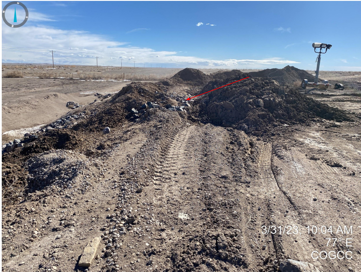
Photo 37. Unconsolidated material placed in front of rip rap portion spillway of sediment basin (red arrow).
