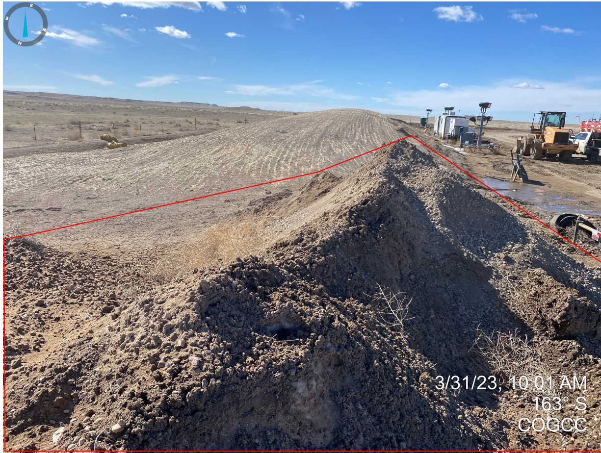
Photo 29. Facing south at the northern end of the location. Unknown material (possibly fill) being stored in close proximity to topsoil stockpile. See comments in Photo 24.
