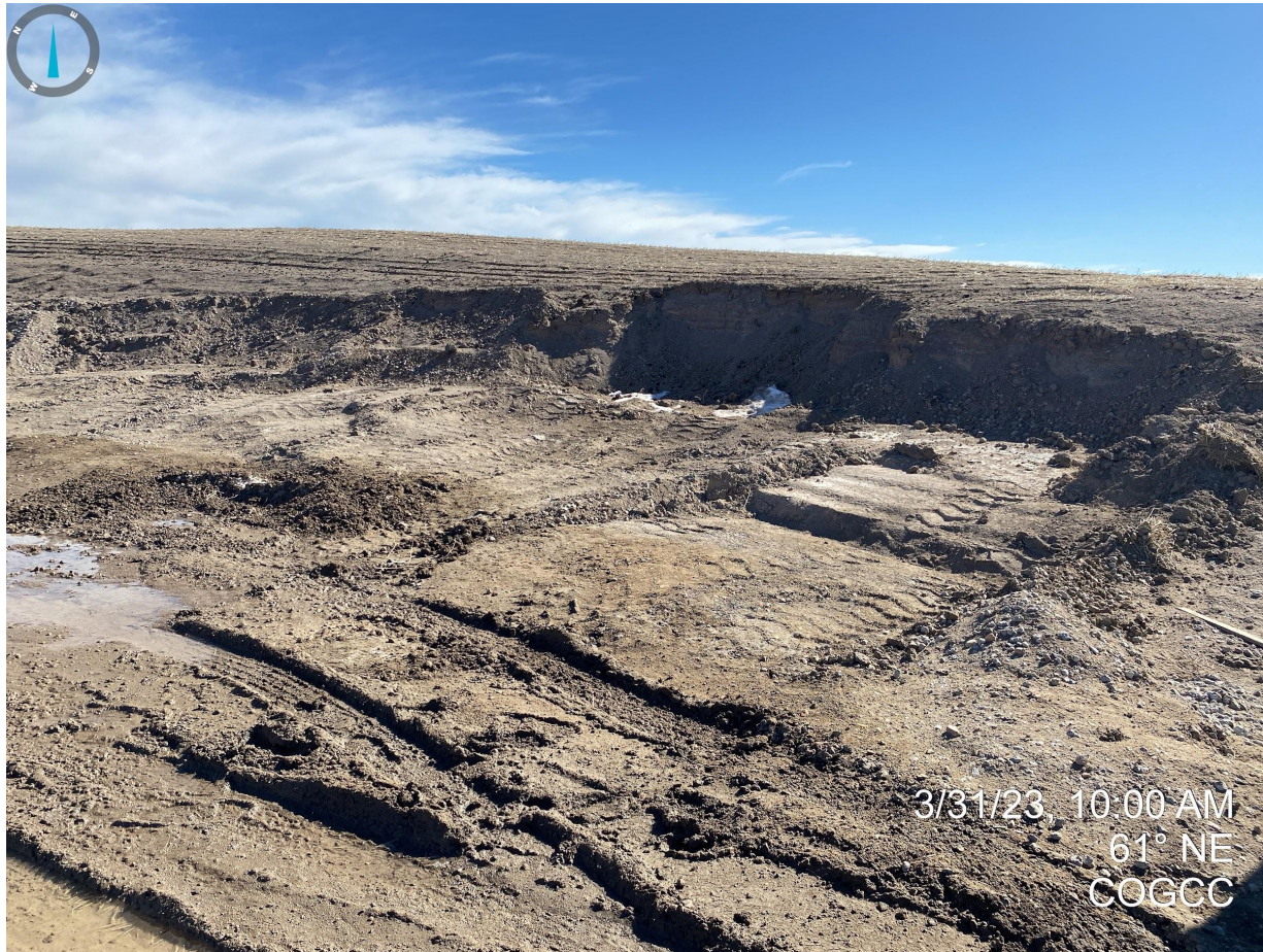
Photo 25. Facing northeast towards topsoil stockpile. It appears an area approximately 40' x 10' x 4' in size has been excavated from the topsoil stockpile. The Operator is being required to import topsoil to replace the deficit.
