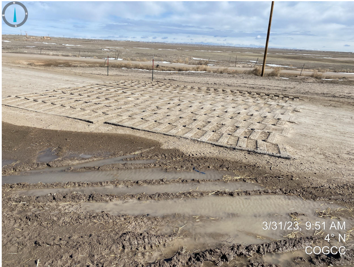
Photo 1. Tracking pad requires maintenance.
