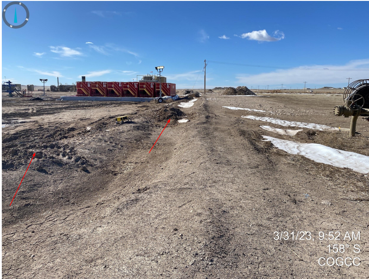
Photo 6. Facing south from the northwest corner of pad. Photo illustrates material in stormwater ditch and unconsolidated material.
