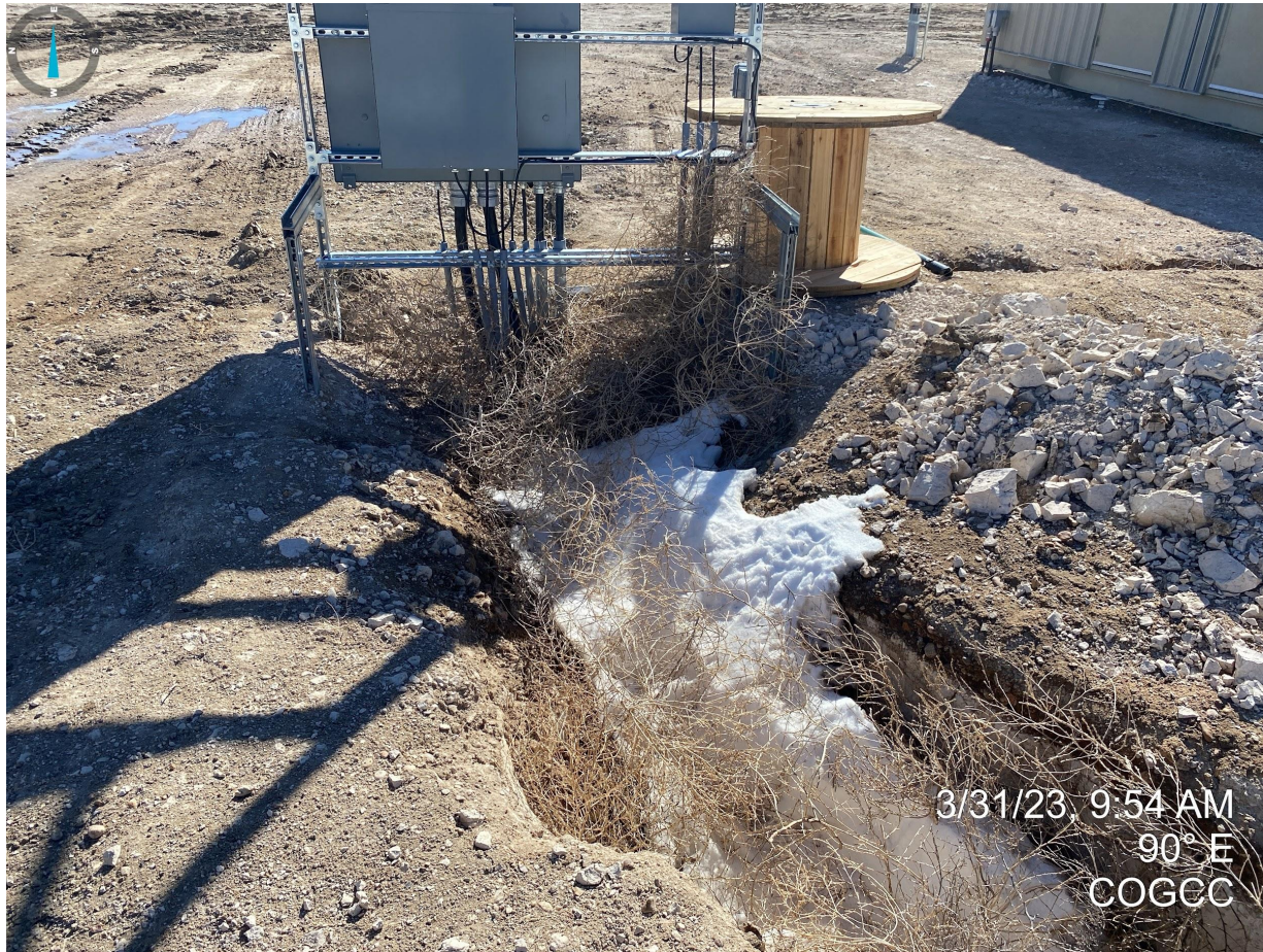
Photo 11. Facing east from southwest corner of pad. Photo illustrates open/subsided trench that hasn't been backfilled or has any type of exclusion device (e.g. construction fence) to prevent injury to personnel or wildlife.
