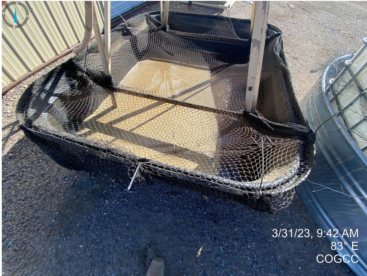
Photo 4. Facing east at raised tank and secondary containment. During this inspection, Staff observed a milky /unknown fluid within the secondary containment that will need to be properly disposed of.
