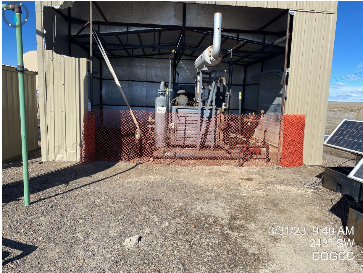
Photo 1. It appears the Operator has performed the corrective action and installed wildlife exclusion device at the entrance of the compressor shed.
