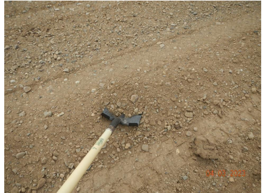
Roadbase loose, not compacted or stabilized, may become new source material in next storm event if no further action taken.
