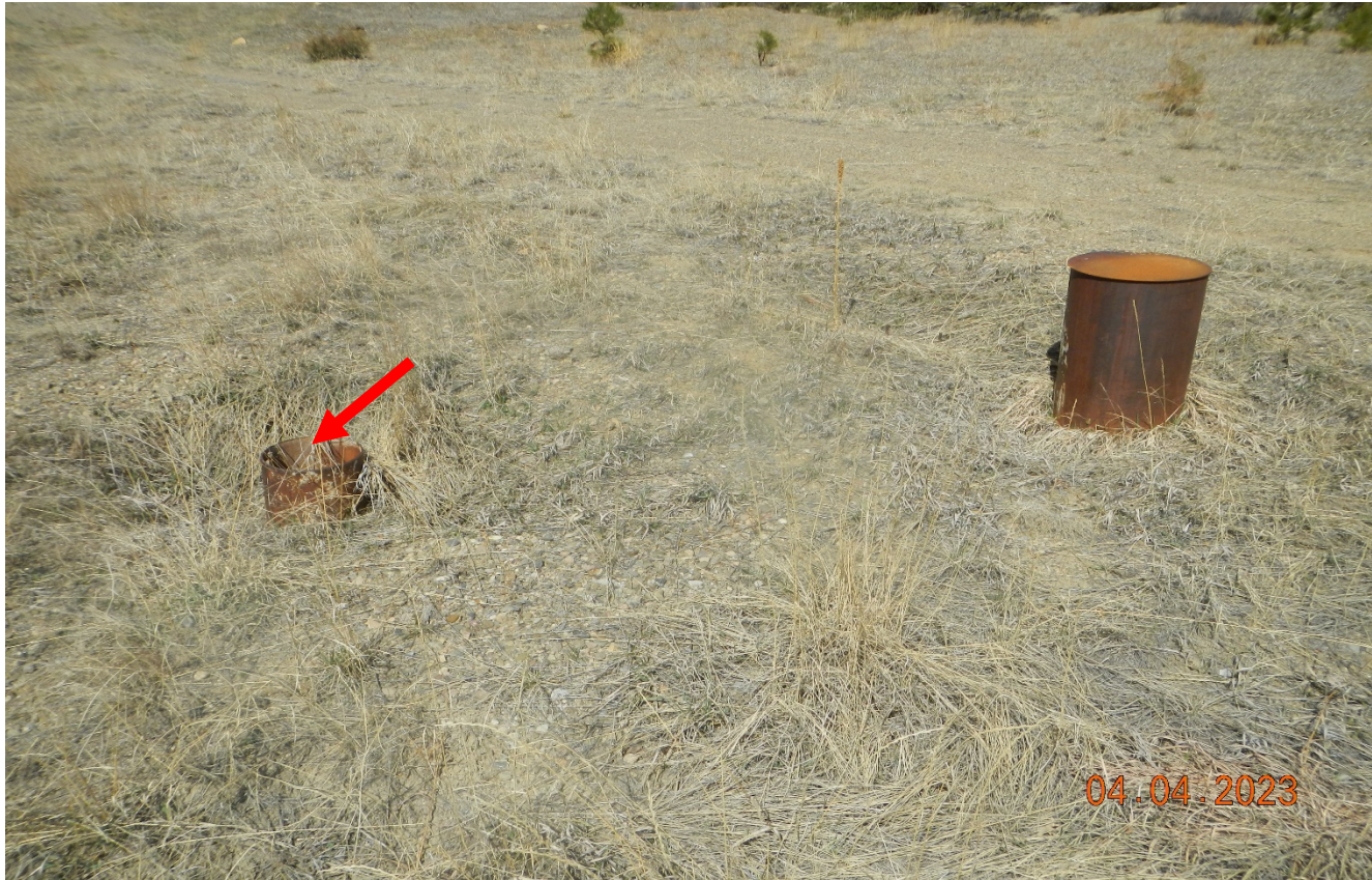
Photo 4. There are 3 steel casings that remain at center of the location. The casing shown at red arrow is not covered to prevent entry. The steel casings need to be removed.
