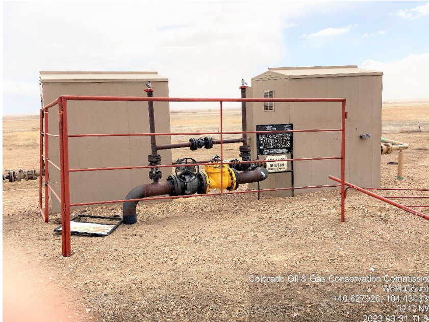
Photo #3 Ball Ranch GW27-63HN Battery site Abandoned: Most Equipment Removed CA: Unnecessary Equipment Gas meter runs, blowdown header
