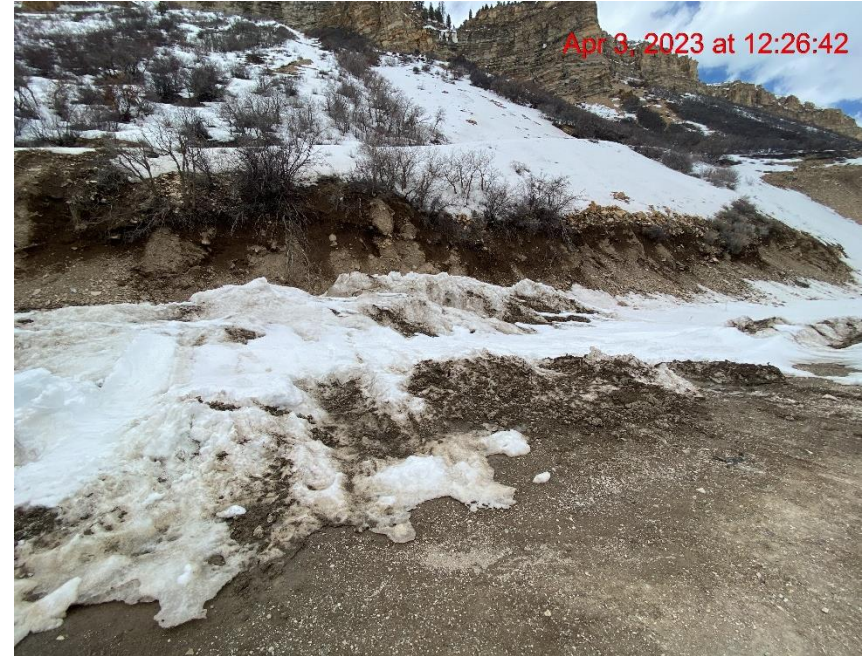
Site: Cut Slope Erosion/Run-On to Location – Photo #01838
