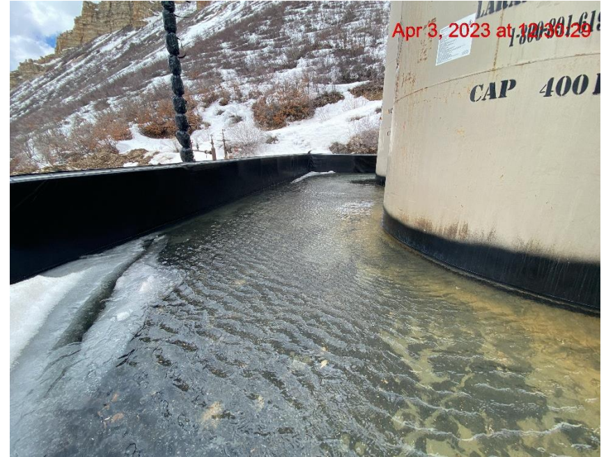
Inadequate Berm Capacity – Photo #01846
