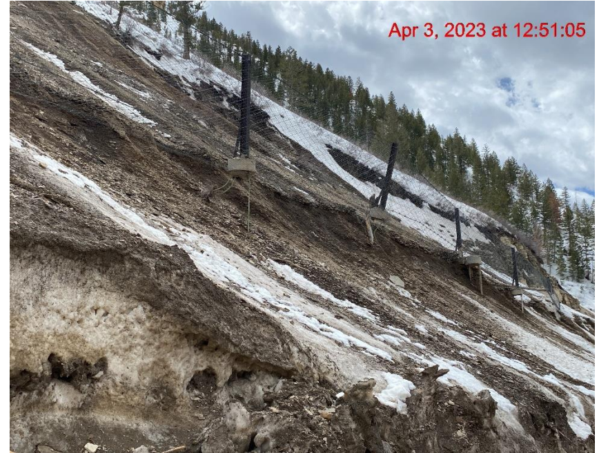
Lease Road: Failed BMP/Slope Erosion/Sediment Migration – Photo #01850
