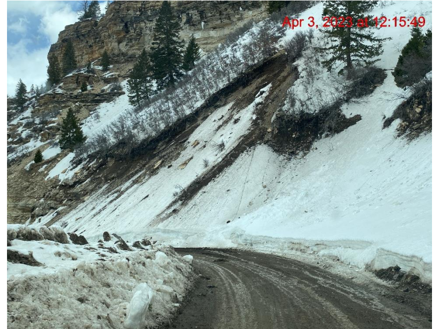
Lease Road: Cut Slope Erosion/Sediment Migration – Photo #01832
