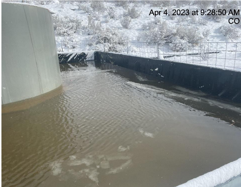
Photo # 4139 Containment capacity inadequate/Failure to maintain containment
