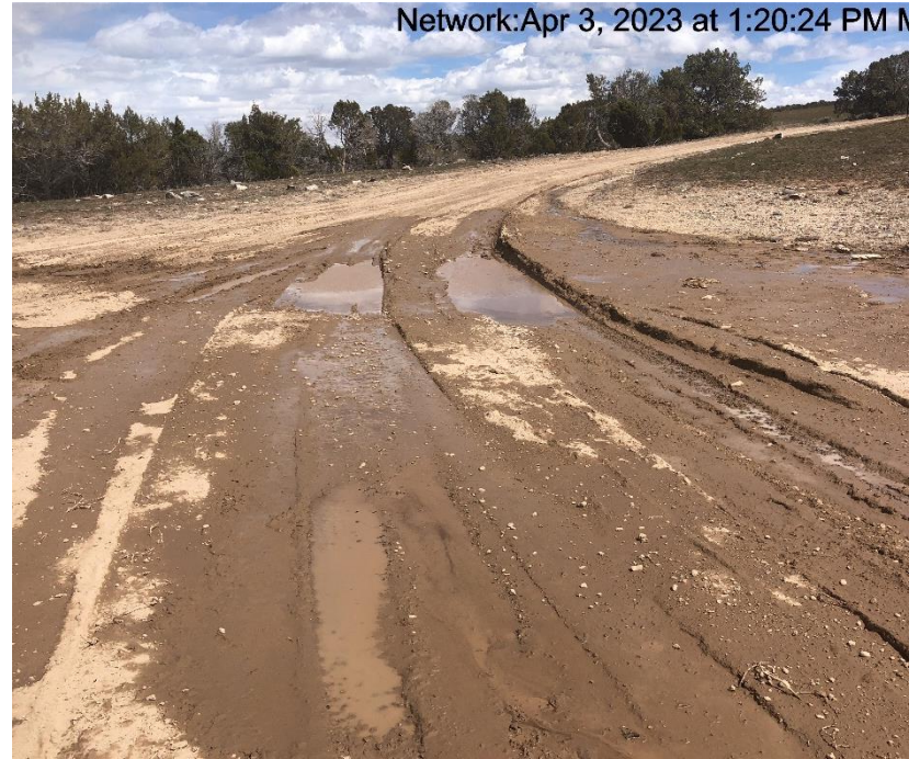
Photo #9525 Insufficient tracking BMP at entrance to location.
