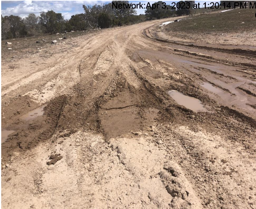
Photo #9524 Insufficient tracking BMP at entrance to location.
