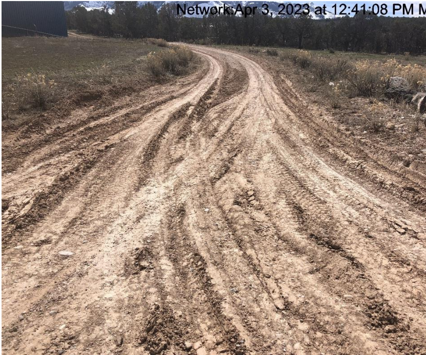
Photo #9486 Insufficient tracking BMP at entrance to location.
