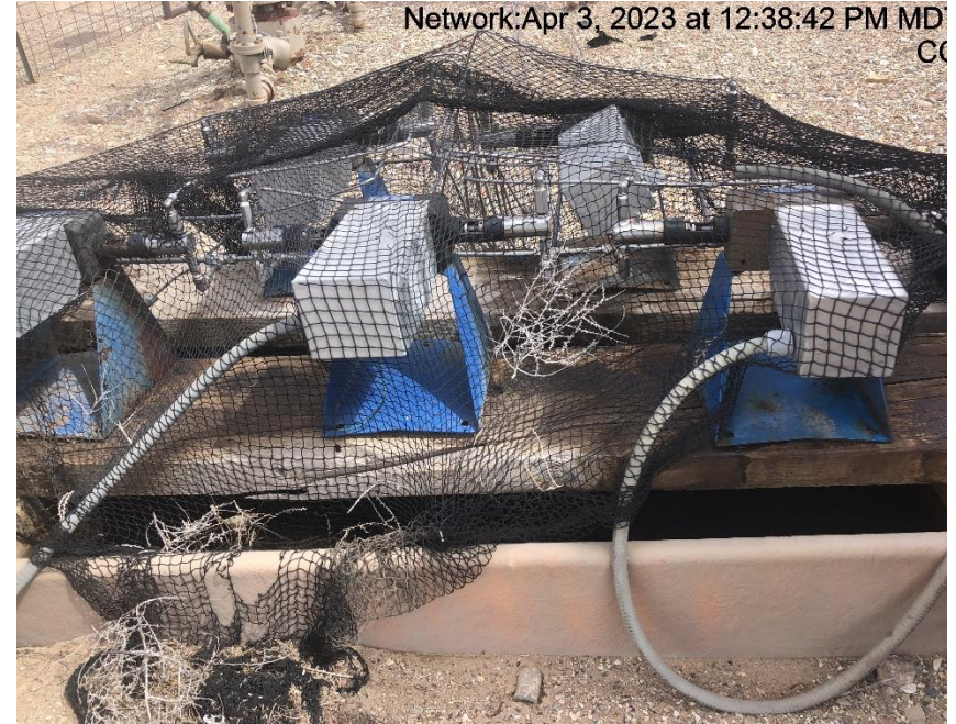
Photo #9479 Bird protector insufficient.
