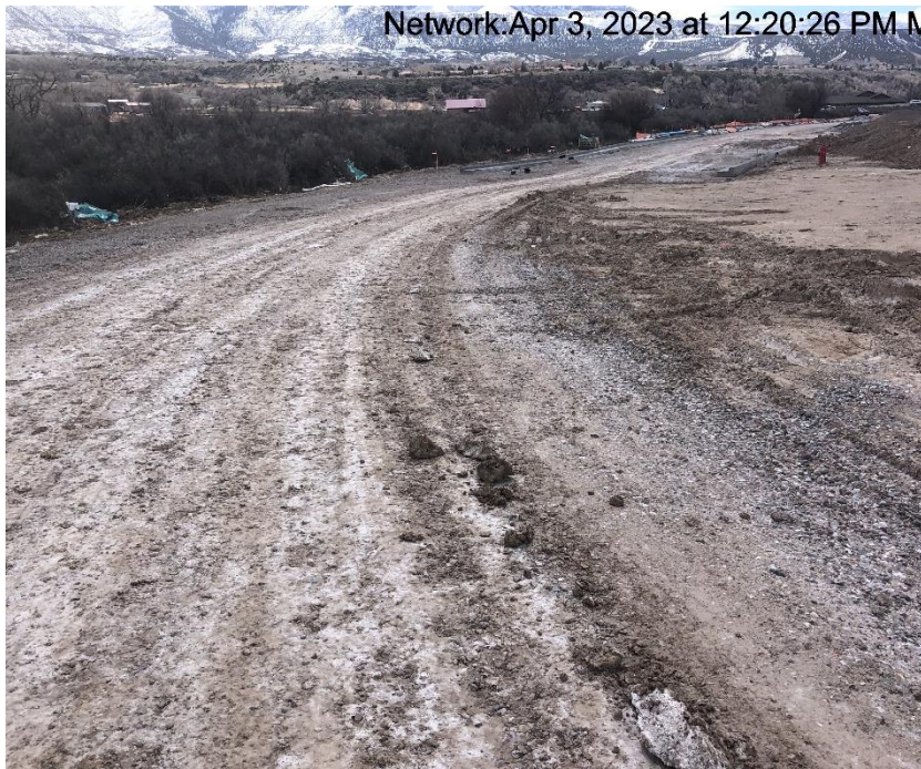
Photo #9472 Insufficient tracking BMP at entrance to location.
