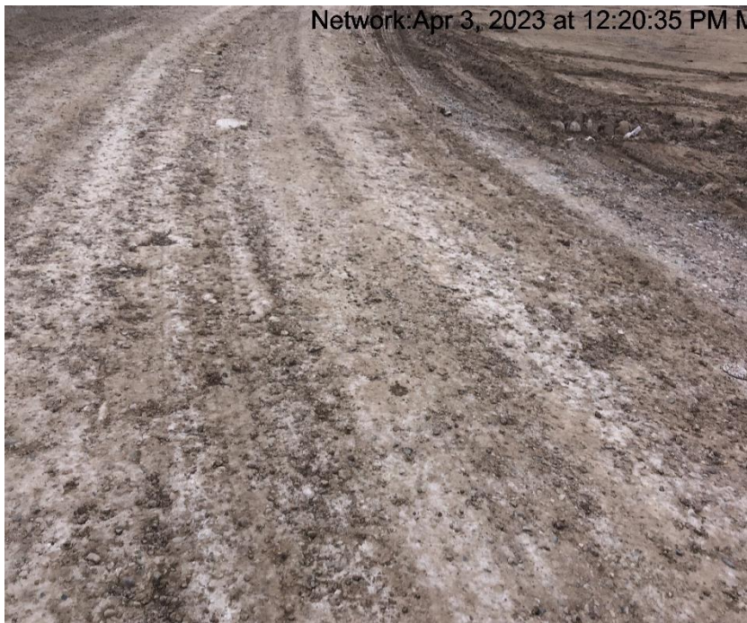
Photo #9473 Insufficient track BMP at entrance to location.
