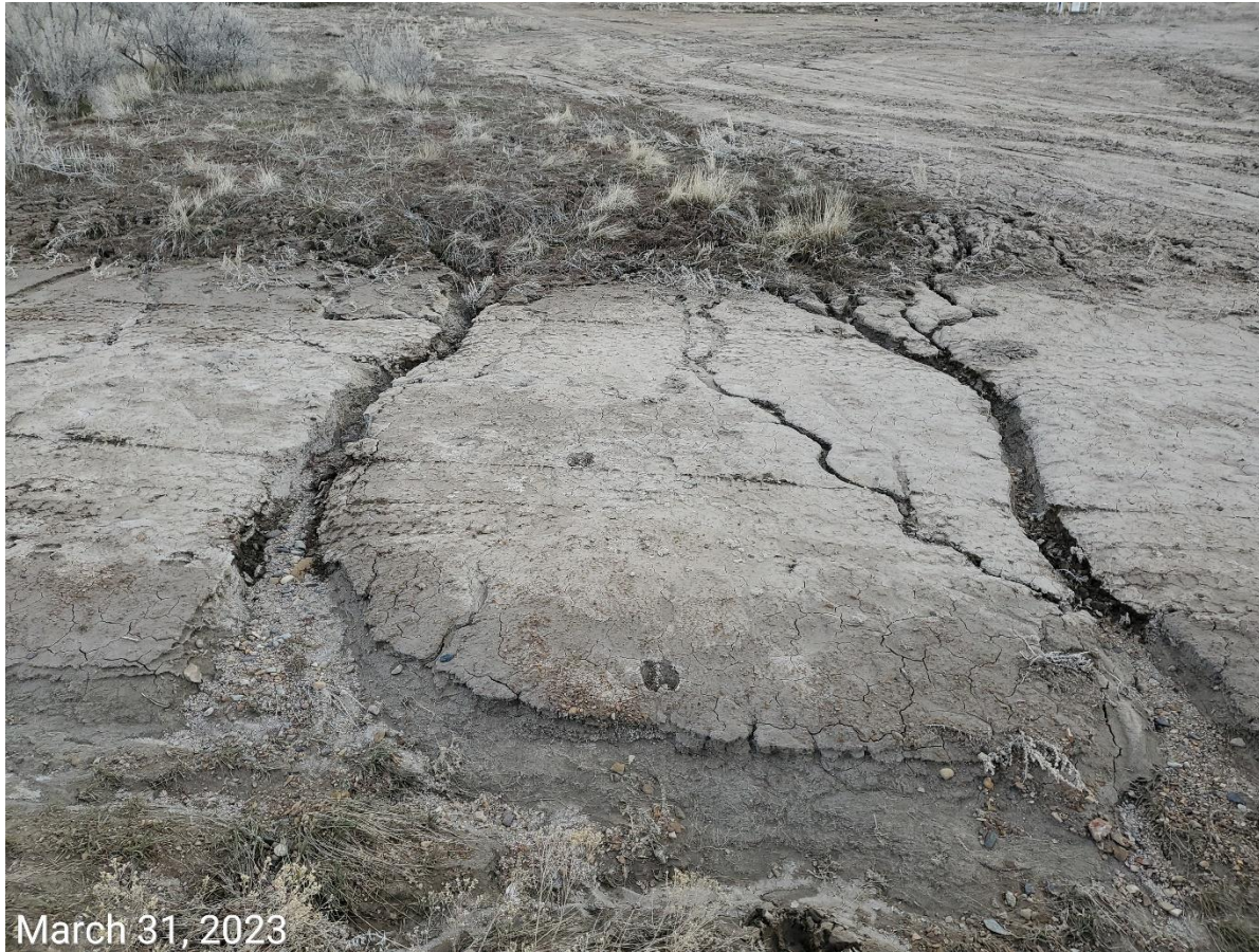
Photo 14: Erosion degradation on access road; stormwater and erosion control BMPs missing or insufficient. Road lacks stabilization.
