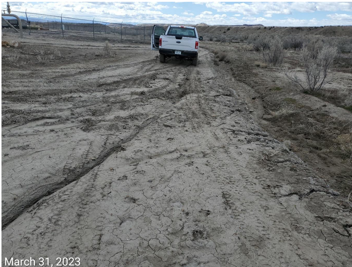
Photo 15: Erosion degradation on access road; tracking controls missing or insufficient; rutting evident. Road lacks stabilization.
