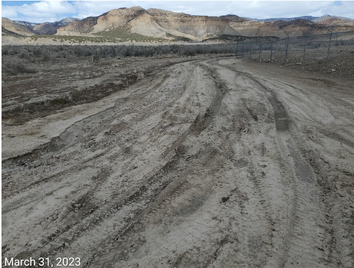
Photo 16: Erosion degradation on access road; tracking controls missing or insufficient; rutting evident. Road lacks stabilization.
