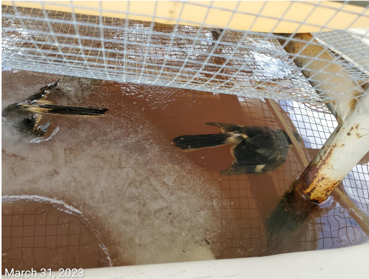
Photo 6: Continued from photo 5. Photo shows wildlife (bird) mortality due to improperly installed/maintain wildlife protection BMPs; bird species observed appears to be Spotted Towhee ( Pipilo maculatus ). Photo also shows containment BMP has filled with fluids, and is not longer adequate to contain a spill.
