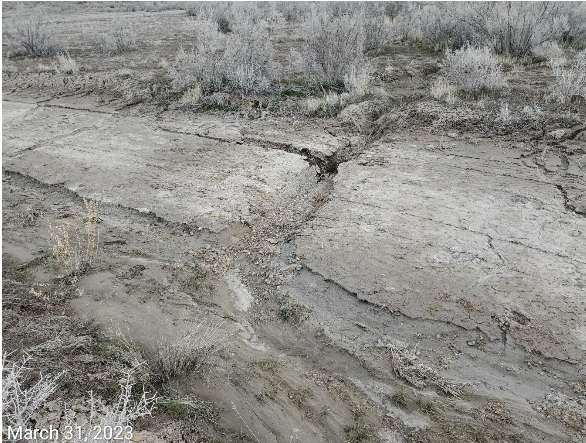
Photo 13: Erosion degradation on access road; stormwater and erosion control BMPs missing or insufficient. Road lacks stabilization.
