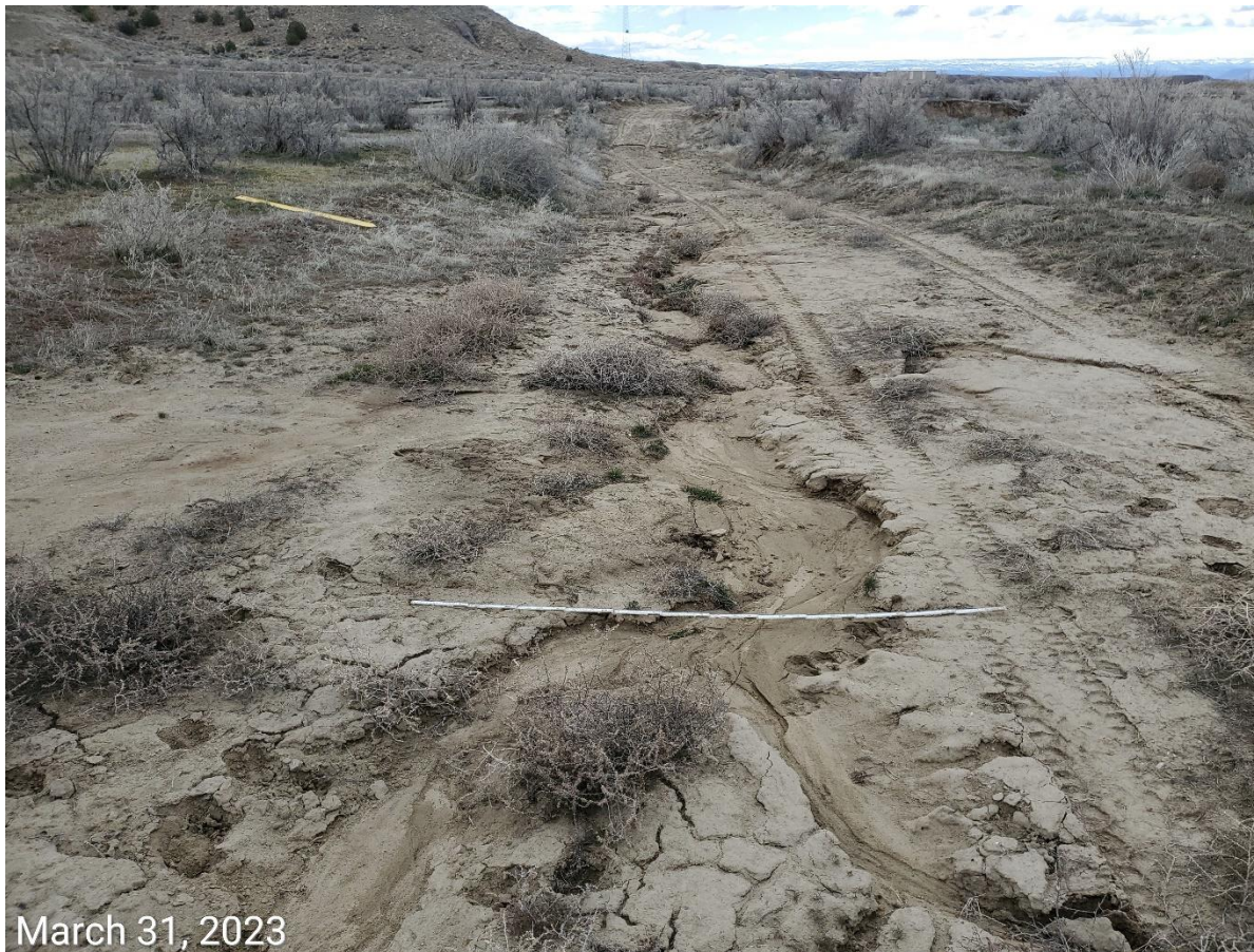
Photo 7: Photo shows erosion degradation due to stormwater runoff on the access road. 6 foot measuring stick for reference. Road lacks stabilization.
