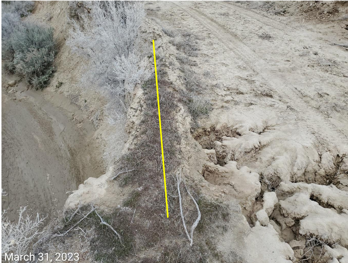
Photo 12: See comments under photo 10. Photo shows areas of access road (right of line) at risk of eroding into Salt Creek (left of line). Road lacks stabilization.
