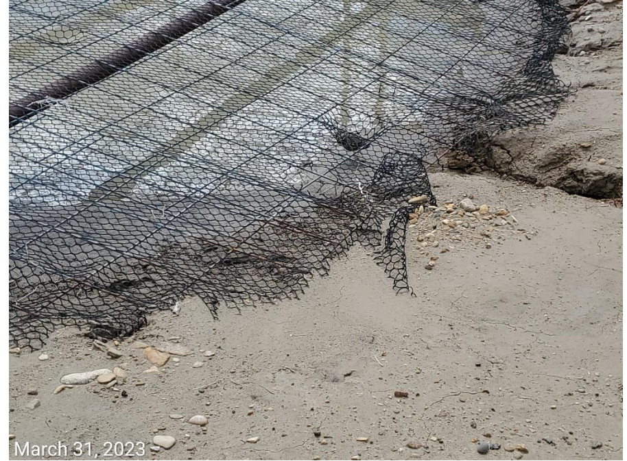
Photo 4: Holes observed in netting at pit; BMP not in proper functioning condition.
