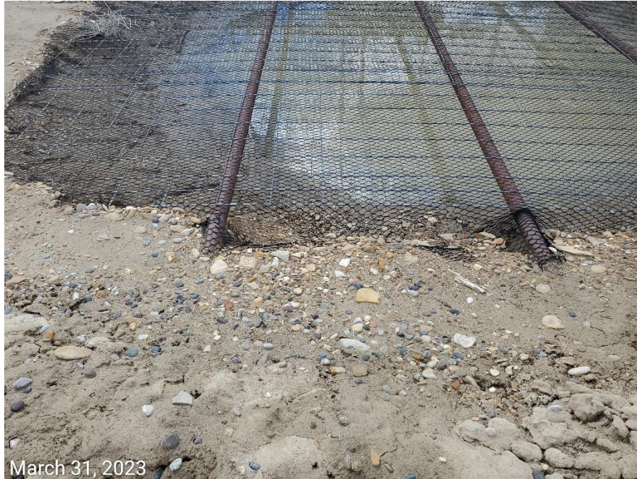
Photo 4: Holes observed in netting at pit; BMP not in proper functioning condition.
