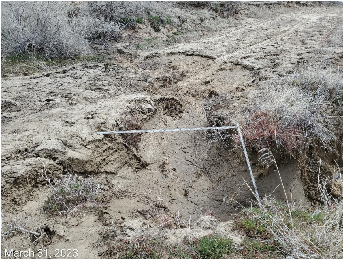
Photo 9: Gully erosion at access road. Photo shows gully depth on that road itself is approximately 2 feet deep. Road lacks stabilization.
