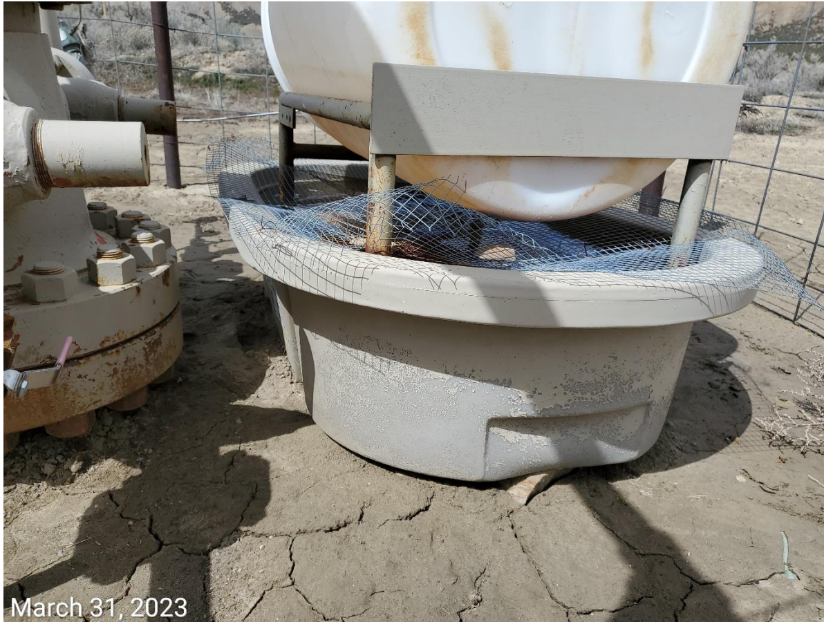
Photo 5: Photo taken from the methanol tank adjacent to the wellhead. Photo shows the wildlife protection BMP (wire fence/net) at the tank has not been properly secured to the containment BMP, which has resulted in bird mortality within the secondary containment.
