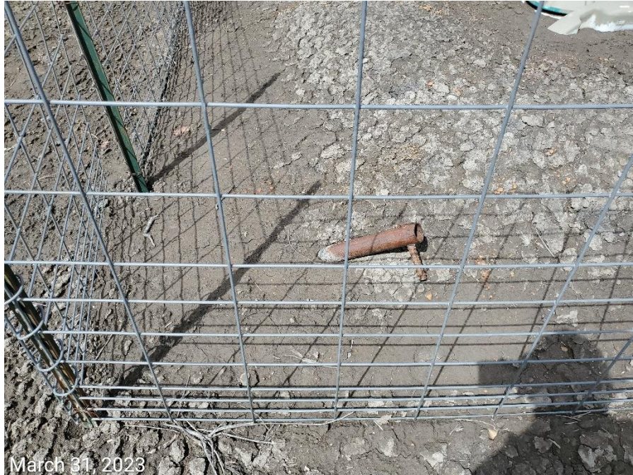
Photo 3: Anchors on location missing required marking.
